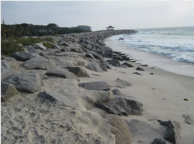
Fort Fisher Revetment
