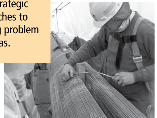
Bridge inspectors examine the strands of a suspension cable.
