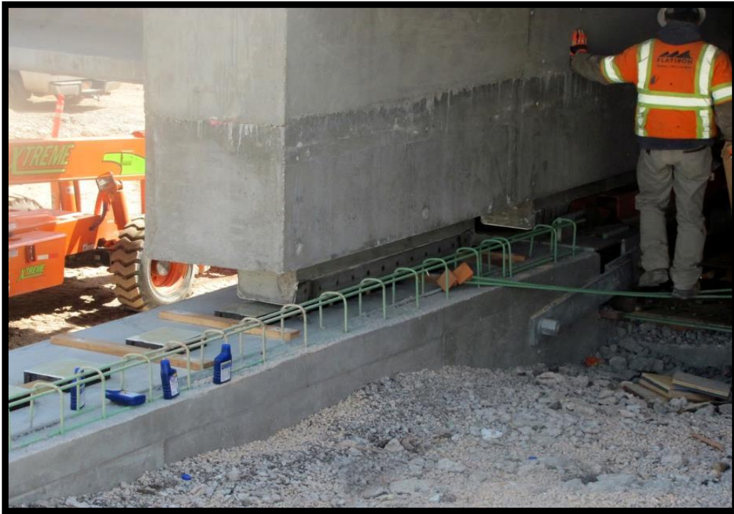
Figure 4-4 Teflon Pads with Stainless Steel Wrapped Shoes on End Diaphragm
