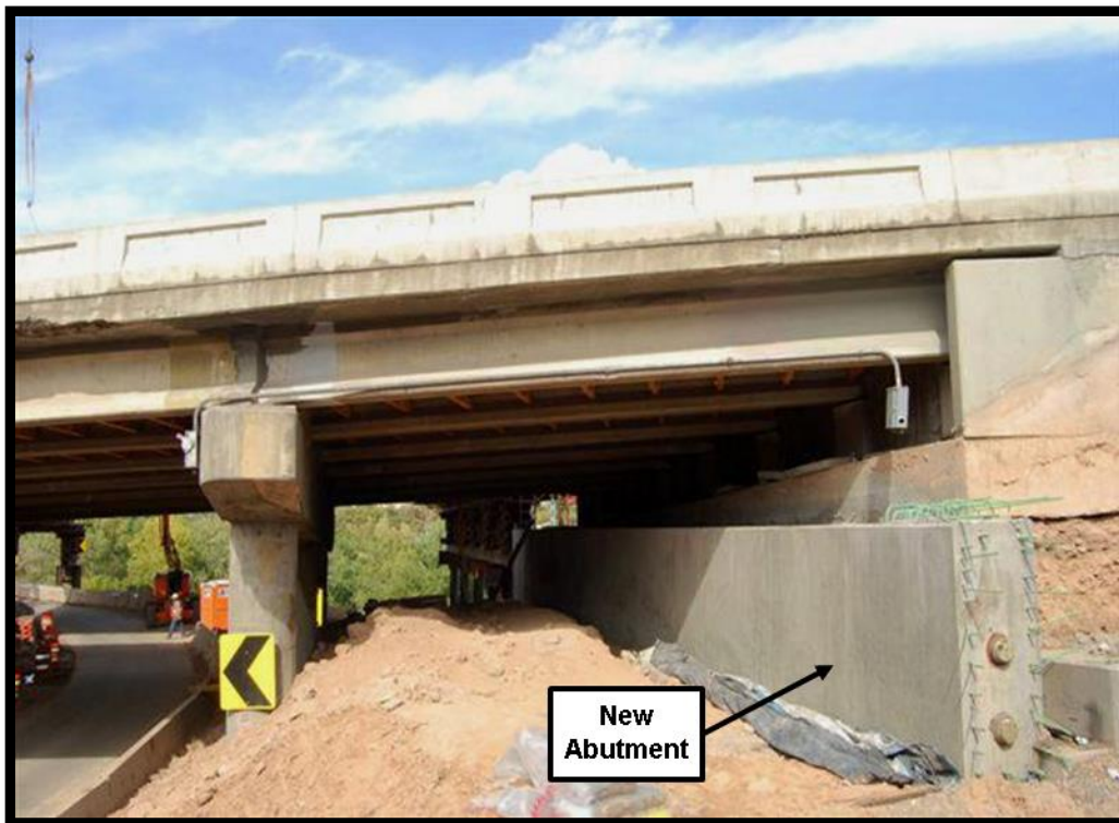
Figure 3-7 New Abutment Constructed under Existing Structure for the I-80; 2300 E. Bridge Slide, Utah
