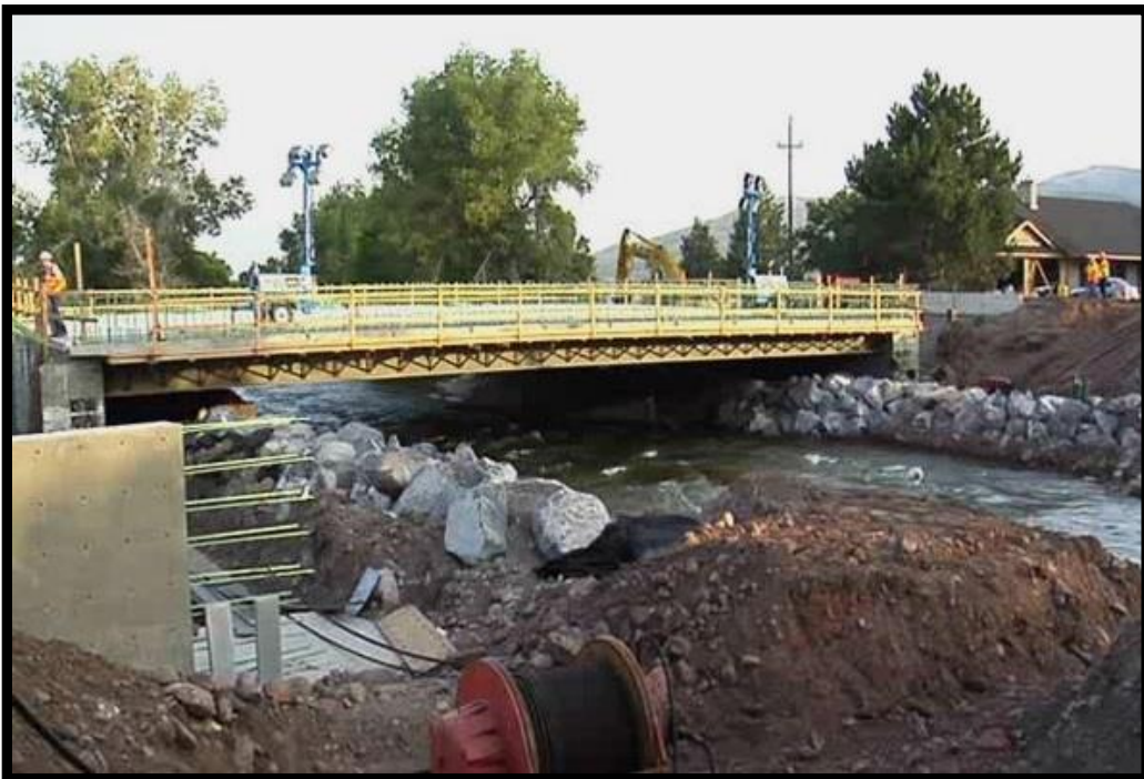
Figure 1-4 SIBC for a Small Stream Crossing for the SR-66 over Weber River Bridge Project, Utah
