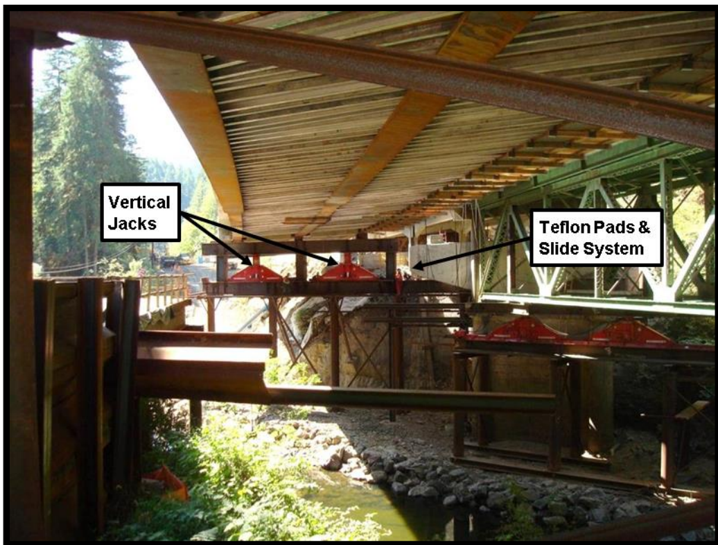
Figure 4-3 Slide Shoes Used with Vertical Jacks
