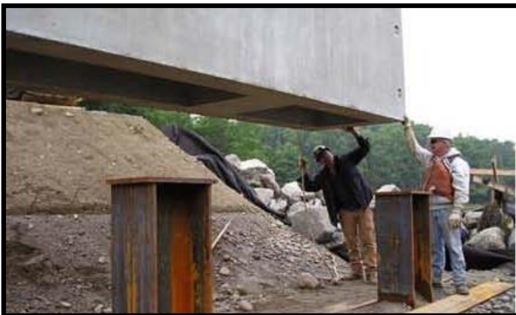
Figure 3-1 Precast Abutment Installation
