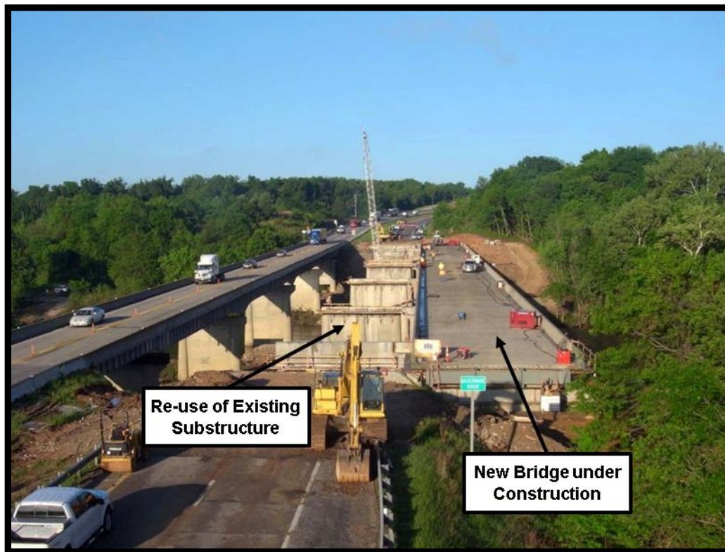
Figure 3-10 SIBC Using Existing Substructure on the I-44 Gasconade River Bridge Project, Missouri
