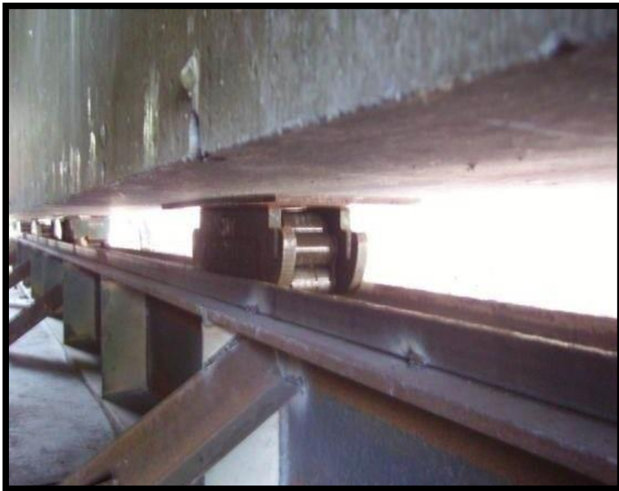
Figure 4-1 Industrial Rollers Used during SIBC
