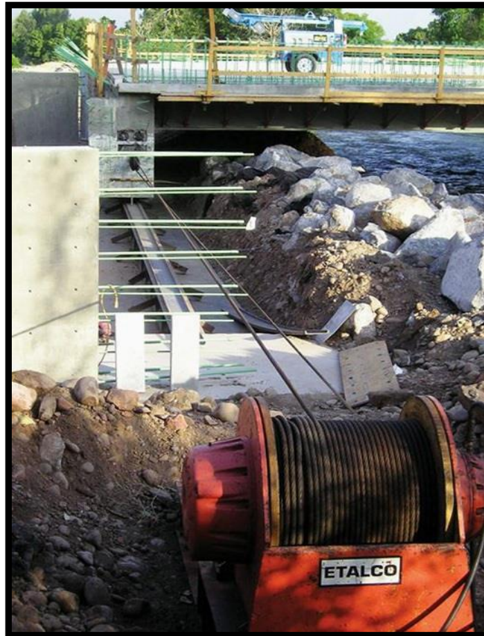
Figure 4-6 Winch System Used to Slide a Bridge over a River
