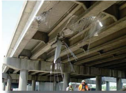
Vertical Underclearance less than current standards
