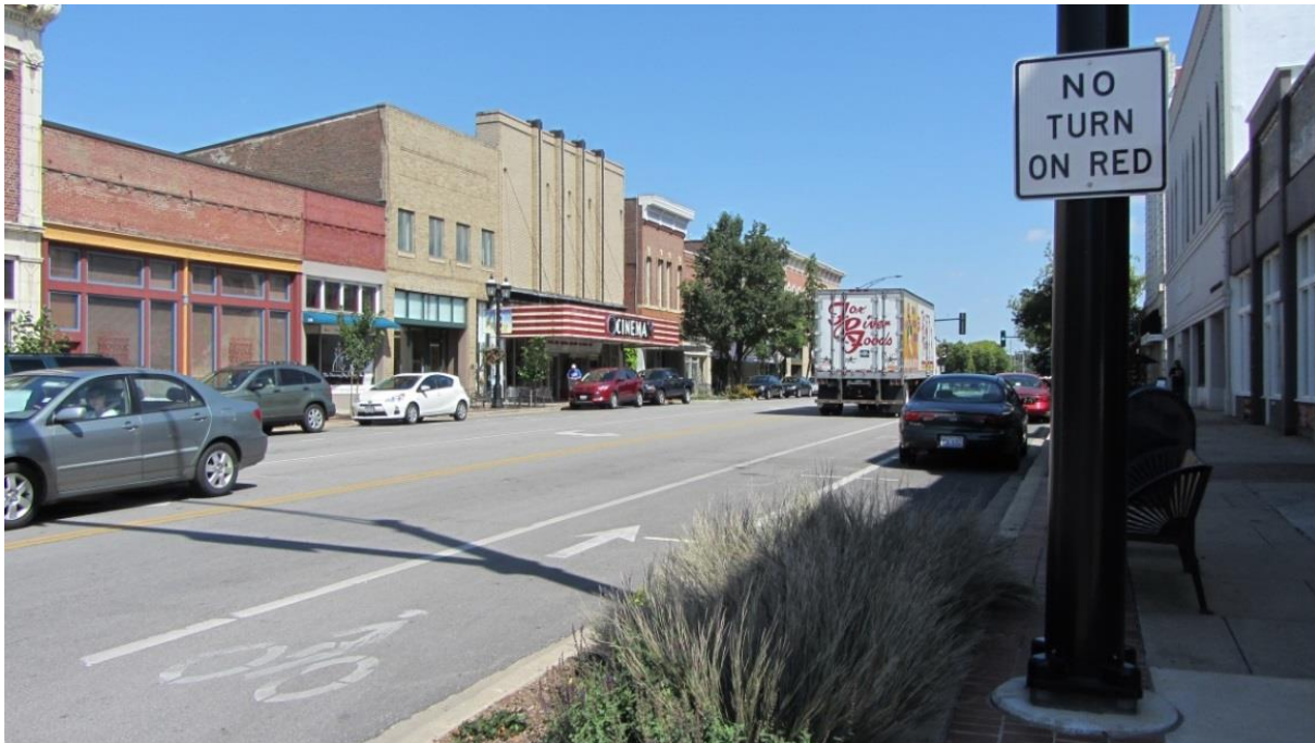
Figure 16. Road diet project on Main Street in Urbana, Illinois. Image courtesy of Champaign County Regional Planning Commission.
