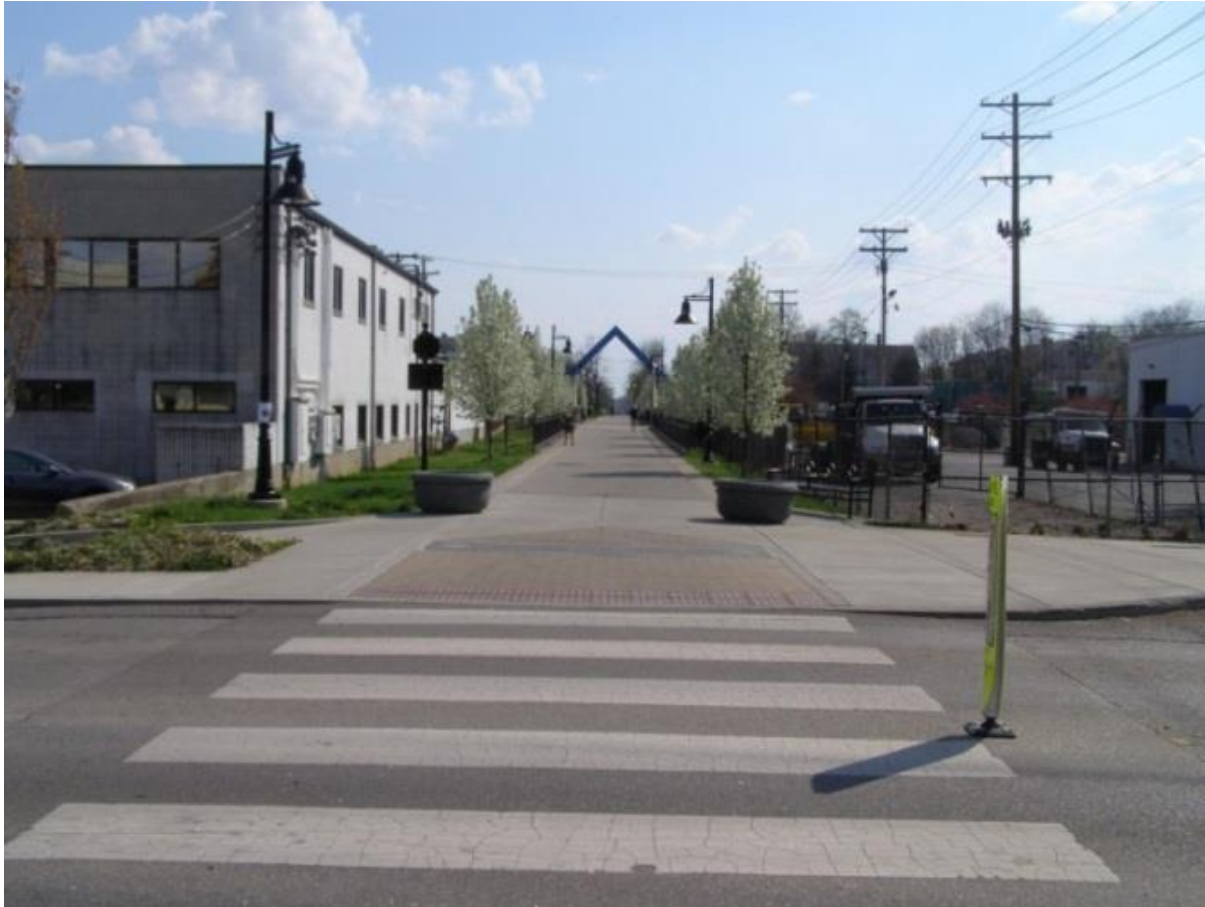
Figure 13. The same rail corridor after the trail was completed. Image courtesy of FHWA Indiana Division Office
