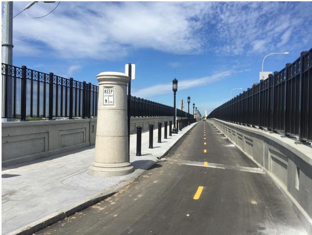
Figure 25. The bridge provides bicycle and pedestrian connections adjacent to the existing I-195 bridge. Image courtesy of Rhode Island DOT.
