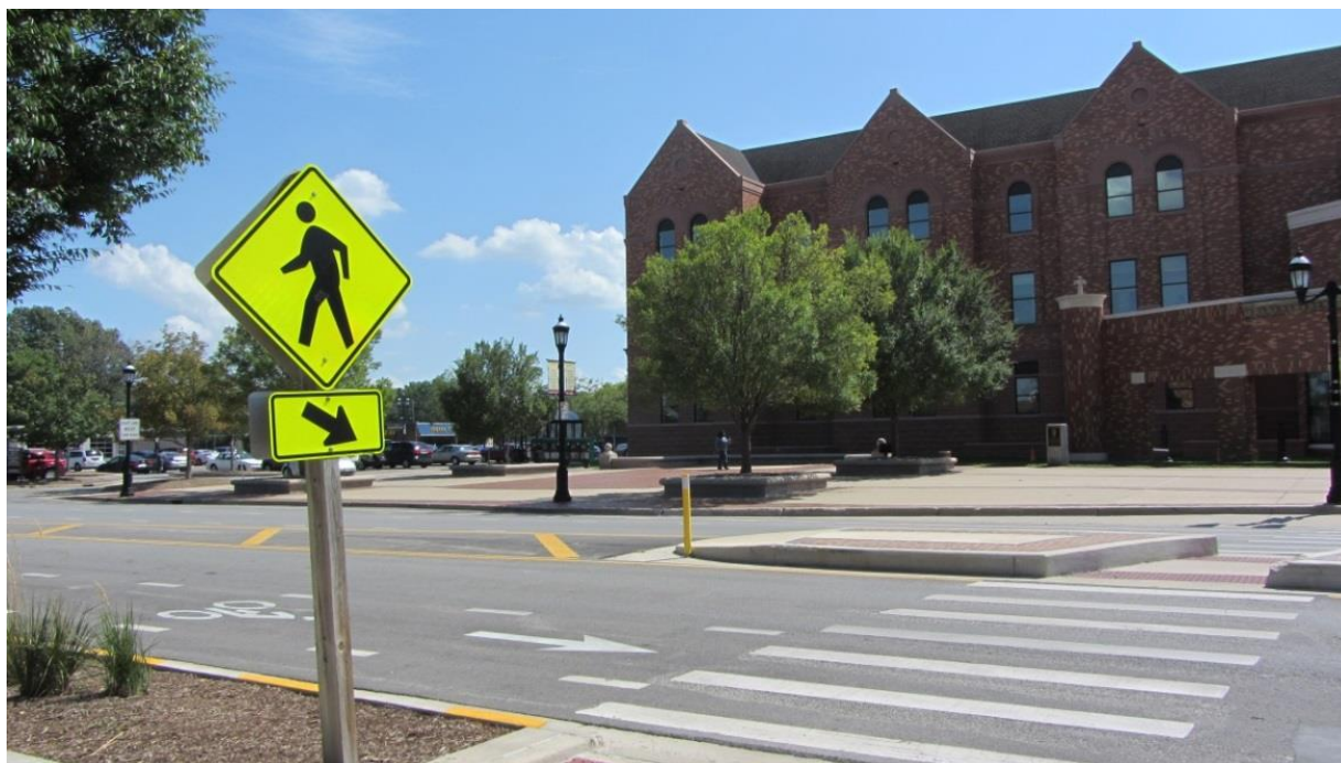
Figure 22. The improvements on Main Street included this pedestrian crossing, complete with a refuge island. Image courtesy of Champaign County Regional Planning Commission.
