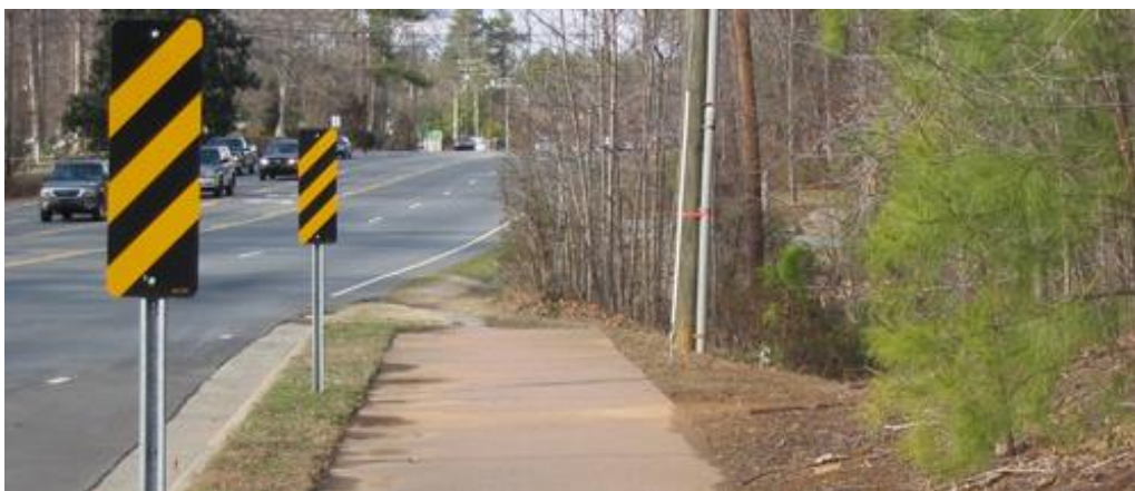
Figure 3. Sidewalks that end abruptly can be significant barriers for individuals with disabilities. Image courtesy of PBIC Image Library (Photographer: Laura Sandt).
