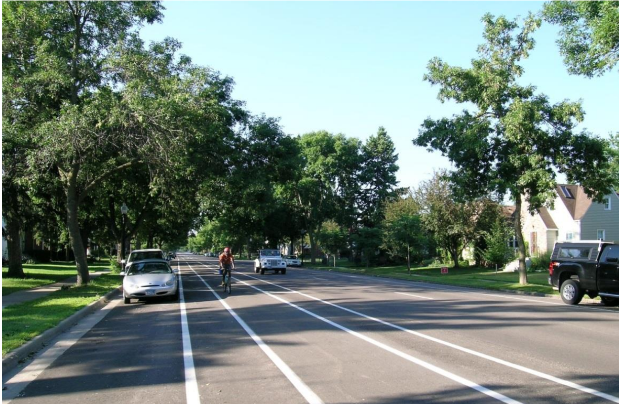
Figure 28. A cyclist riding in the buffered bicycle lane. Image courtesy of the FHWA Minnesota Division Office
