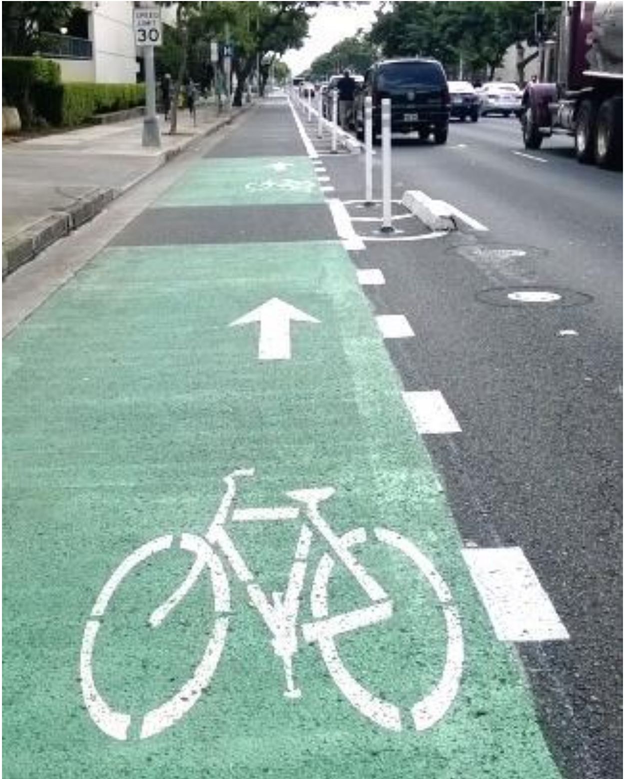
Figure 30. The green buffered bicycle lane with a buffer separating it from the travel lane. Image courtesy of HDOT.
