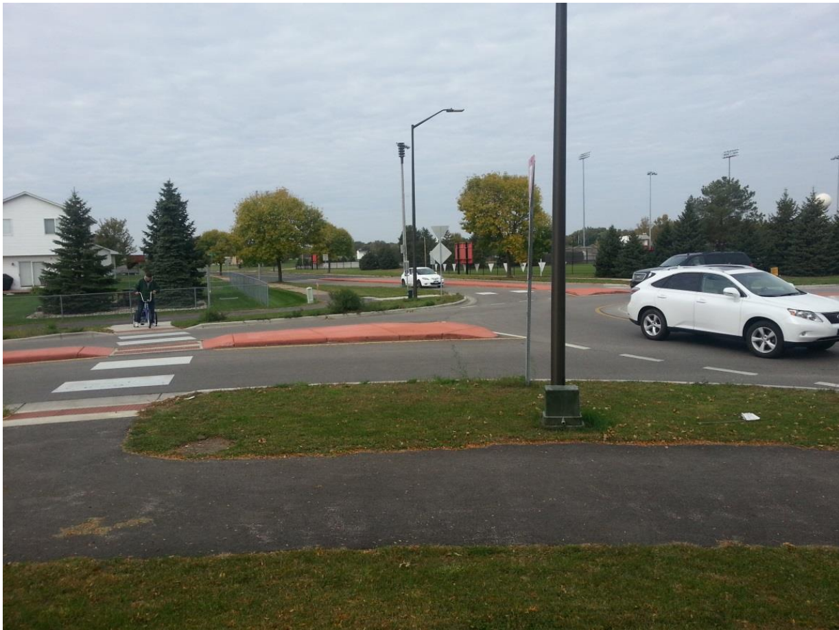
Figure 32. The final result of the intersection conversion to a roundabout. Image courtesy of the FHWA Minnesota Division Office.
