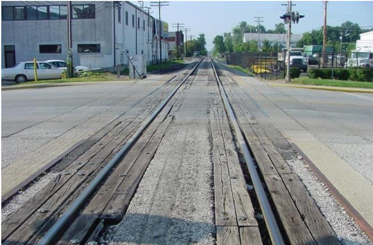
Figure 12. The abandoned rail corridor through Bloomington that was selected for the B-Line Trail development. Image courtesy of FHWA Indiana Division Office.
