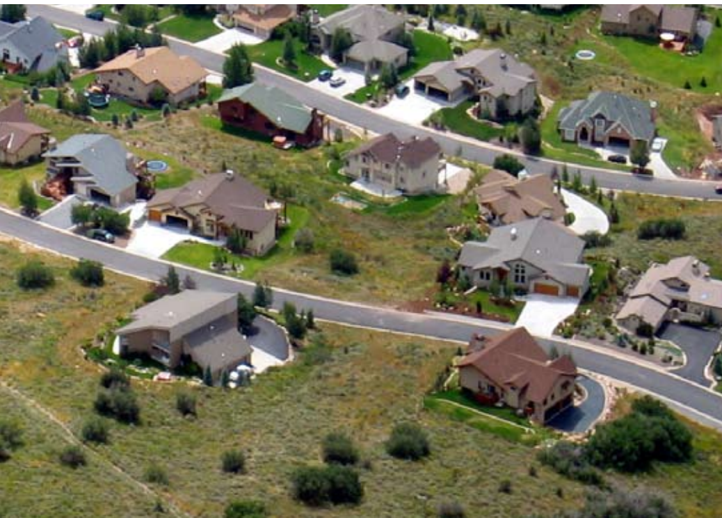
HOME-TO-HOME IGNITION, AS A RESULT OF BURNING EMBERS, CONTRIBUTED TO THE DEVASTATION IN THIS SAN DIEGO, CALIF., NEIGHBORHOOD AS A RESULT OF THE WITCH CREEK WILDFIRE IN OCTOBER 2007.
