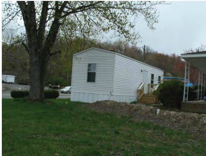
A temporary housing unit on a private property site. Source: OIG
