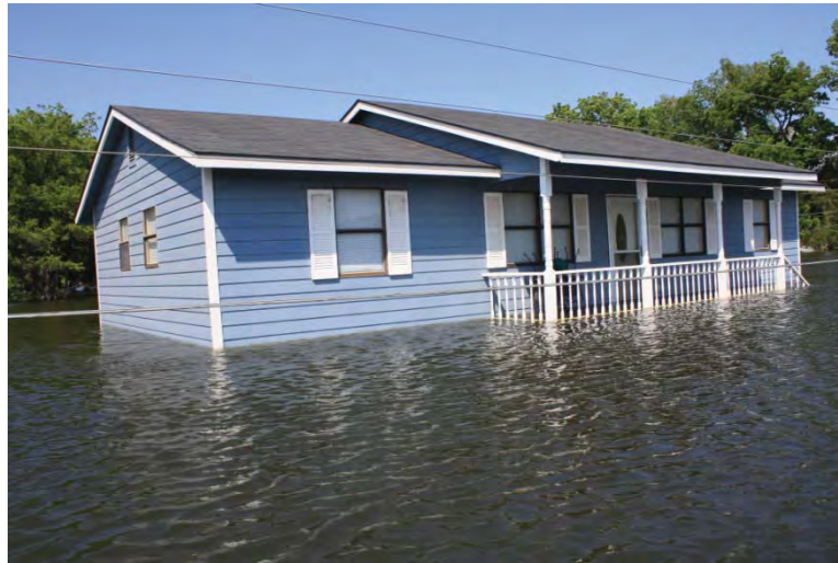
The rising waters of the Mississippi River surround this home in Vicksburg, MS. Source: FEMA
