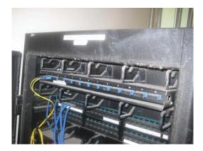
Figure 6- Dust covered Sensitive Equipment
