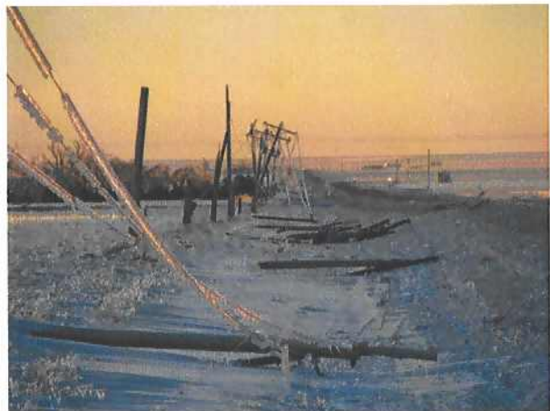
Downed utility poles due to ice-loaded utility lines
