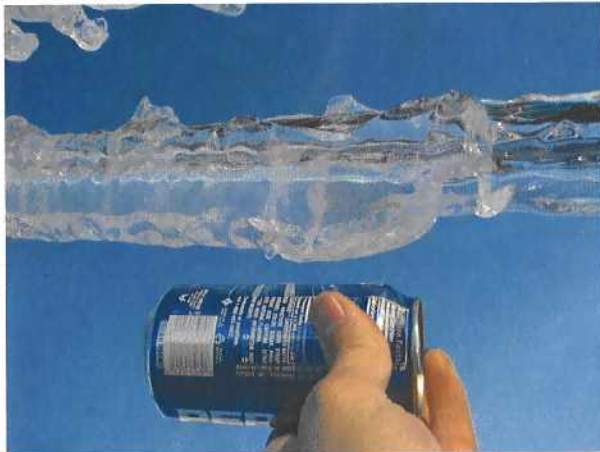
Ice-loaded utility line Source: PEC officials
