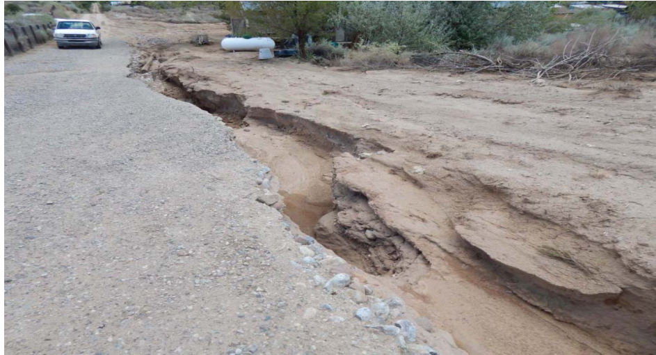
Figure 1. Damage to Hollywood Road after flooding in DR-4148
