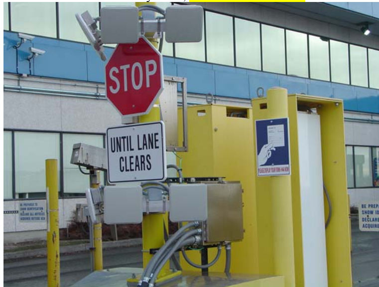
Picture 1 – US-VISIT Entry Lane, -----
