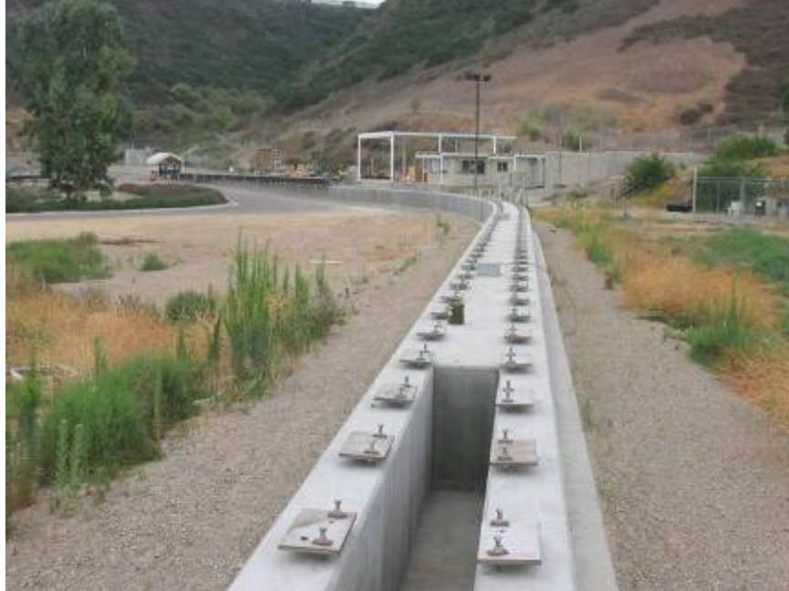
Figure 3.2-8 View from North end of track, showing “maintenance pit” and in the distance the straight guideway modules 1, 2, and 3
