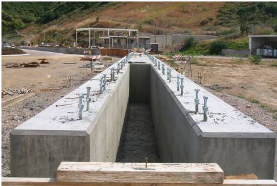
Figure 3.1-5 Cut-out in segment F-8 for vehicle service access
