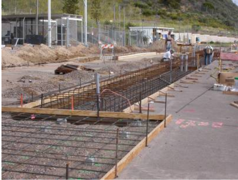
Figure 3.1-2 Set-up patio (F-9) and segment F-1 formwork and rebar installed
