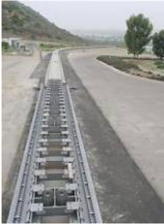
Figure 1-4 Completed 120-m test track foundation, and first 15-m guideway weldment (left). Right picture shows completed guideway module ready for turning over
