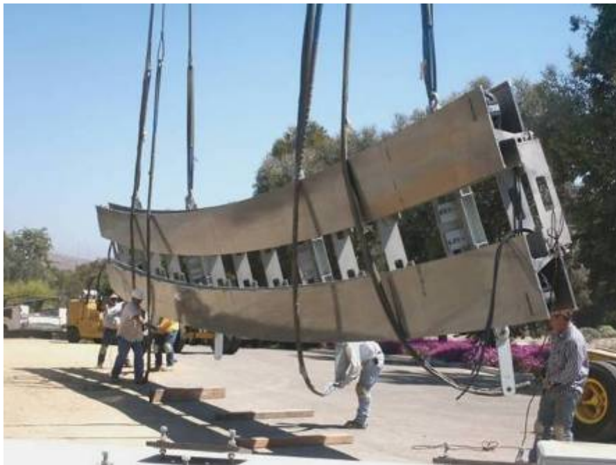
Figure 3.2-9 Curved guideway module being installed on the foundation
