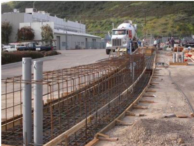
Figure 3.1-3 South spiral (F-4) foundation slab and pedestal rebar installed
