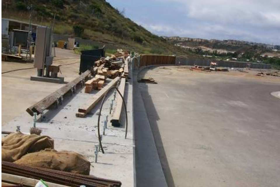
Figure 3.1-6 All segments F-1 thru F-8 and F-9 south set-up patio completed
