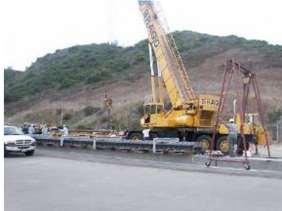
Figure 1-4 Completed 120-m test track foundation, and first 15-m guideway weldment (left). Right picture shows completed guideway module ready for turning over
