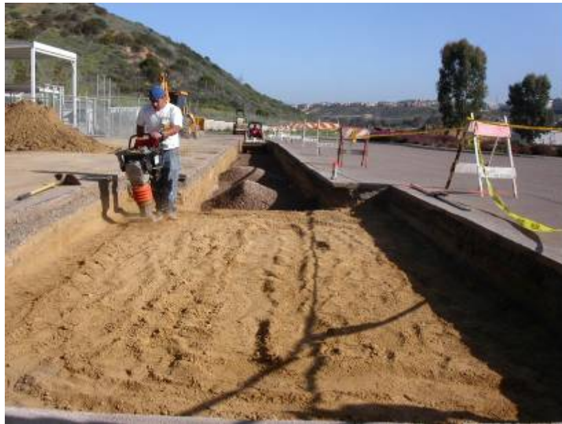
Figure 3.1-1 Foundation excavation and compaction in progress
