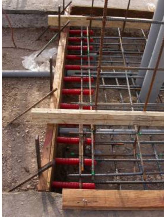
Figure 3.1-4 Typical slab segment separation expansion joint
