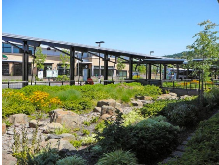
Figure 3-17 Bioswale at Springfield Station
