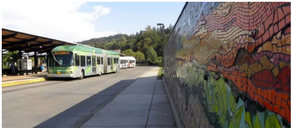
Figure 3-5 Glass mosaic wall at Springfield Station
