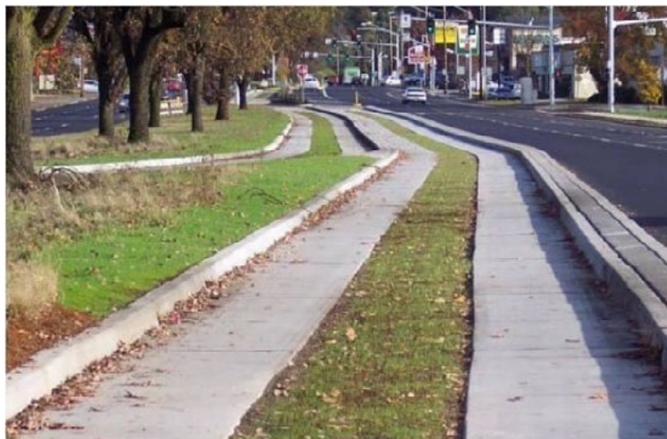
Figure 3-13 Grass strip in center of Franklin EmX running way
