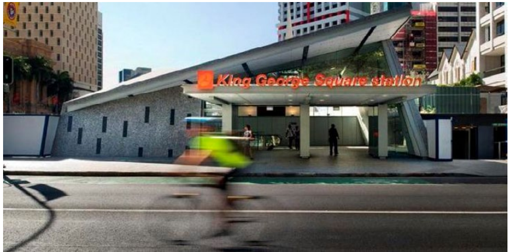
Figure D-9 King George Square Station, Brisbane
