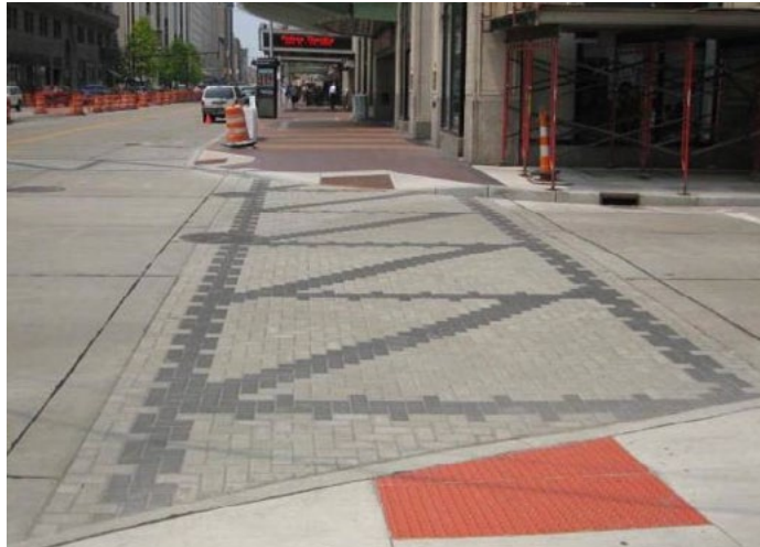
Figure 4-15 Downtown crosswalk paved in concrete brick pattern
