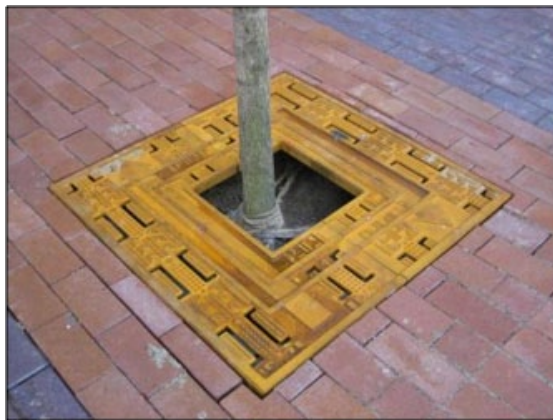
Figure 4-8 Cast iron decorative tree grate and rendered granite sidewalk art
