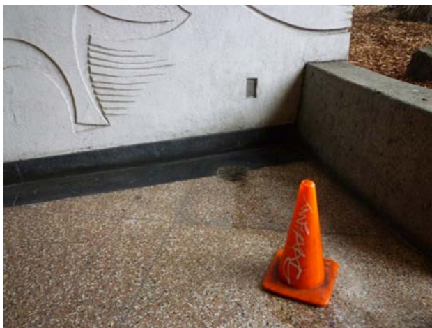
Figure 3-4 Inlet near Fountain
