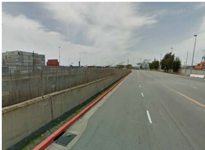
Figure 3-8 Storm Drain Inlet in Street near Oakland West Portal
