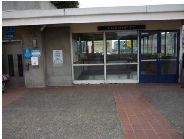
Figure 3-2 Station Stair and Elevator Entrance
