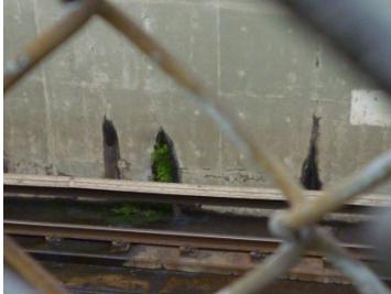
Figures from left-right: Plants growing in retaining wall cracks, gate along 7 th St, track portal looking east.
