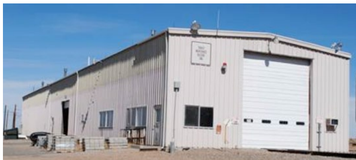
Transit Maintenance Building (TMB)
