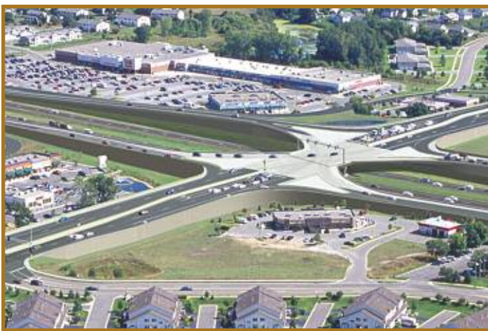
Through an extensive public involvement and outreach process the TH 65-CSAH 14 interchange improvement project met its goal of maximizing safety, capacity, and mobility, while minimizing disruption to the local businesses and residents.
