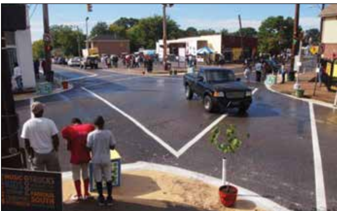
Figure 7: MemFix Temporary Intersection Improvements, Including Crosswalk Markings and Curb “Bulbouts” to Provide Safer Spaces for Pedestrians Waiting to Cross.
