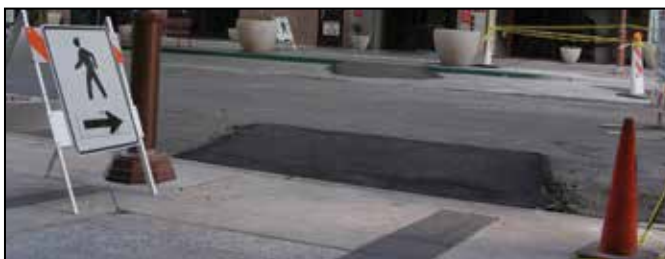
A Stable, Temporary Curb Ramp
