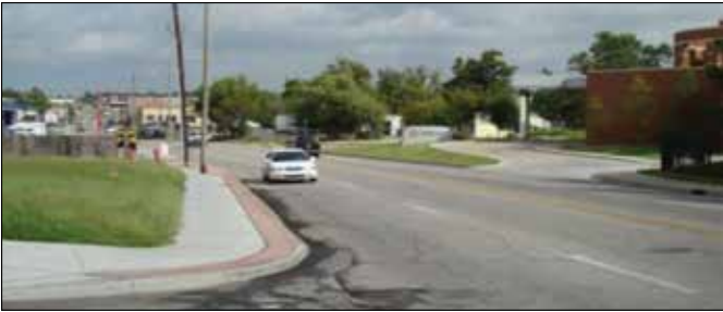
Figure 5: New Sidewalk Along Utica Avenue.
