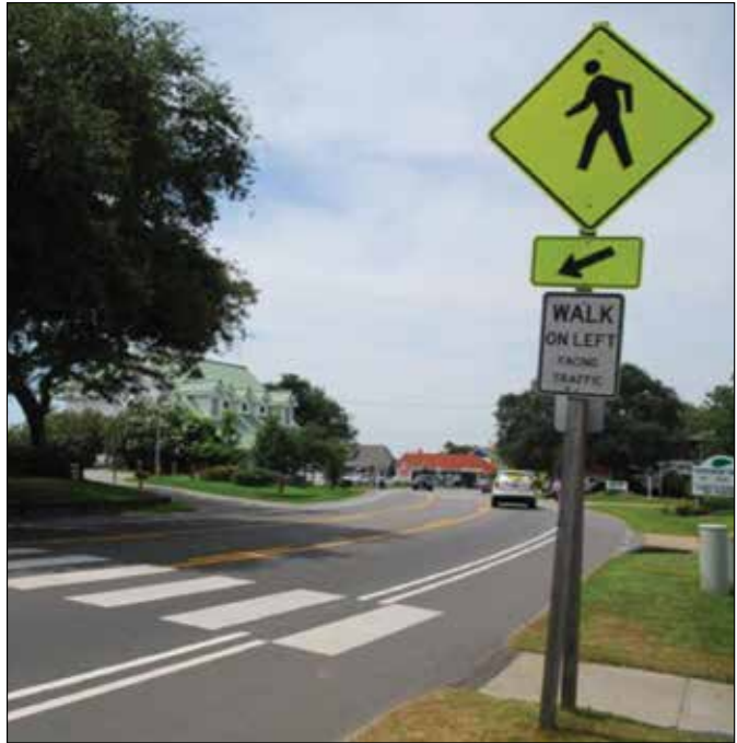
Figure 3: Crossing Improvements Included Pavement Markings and Signage for Drivers and Pedestrians at Crosswalks.
