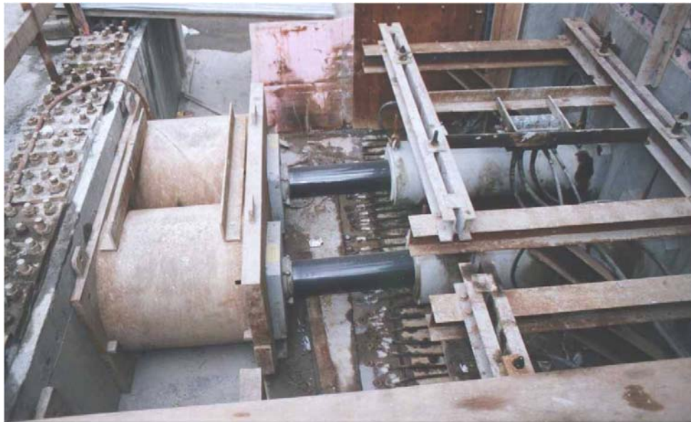
Figure 12-7 Close Up of High Capacity Hydraulic Jacks, Reaction Blocks, and Packers
