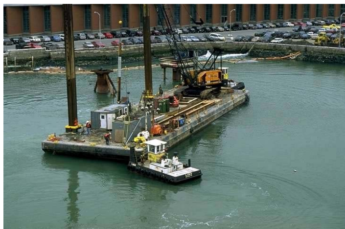
Figure 11-9 Fort Point Channel Tunnel, Boston
