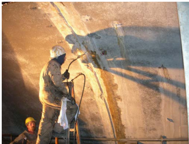
Figure 16-4 Leak Injection, Tuscarora Tunnel PA Turnpike
