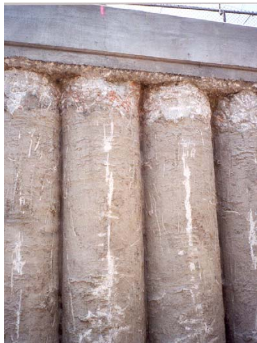
Figure 5-8 Tangent Pile Wall Construction Schematic
