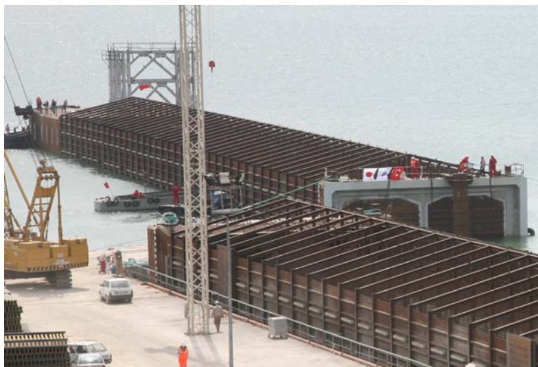
Figure 11-8 Bosphorus Tunnel, Istanbul, Turkey
