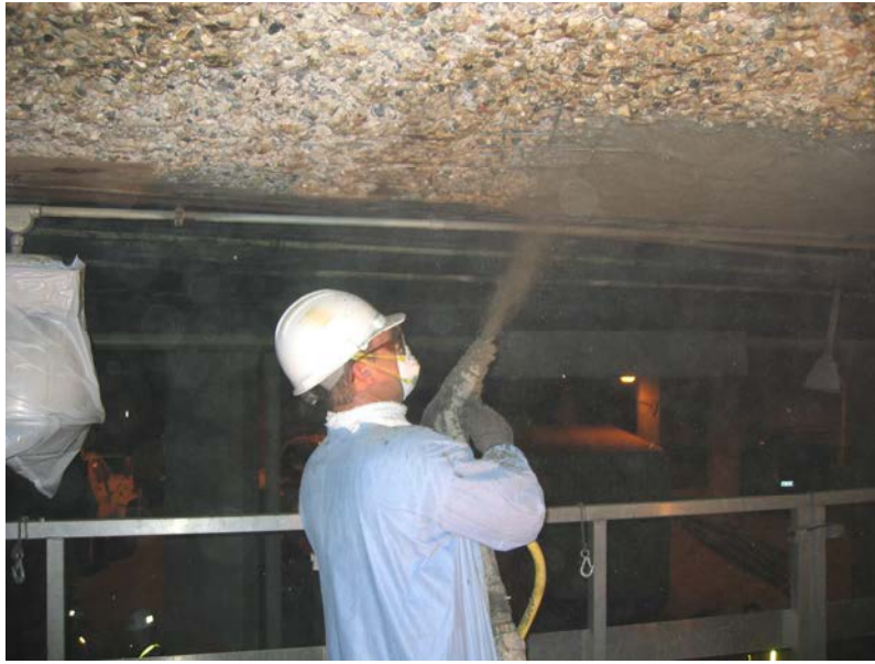
Figure 16-11 Nozzleman Applying Wet Process Shotcrete, USPS Tunnel Chicago
