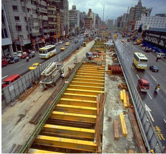
Figure 5-7 Braced Slurry Walls
