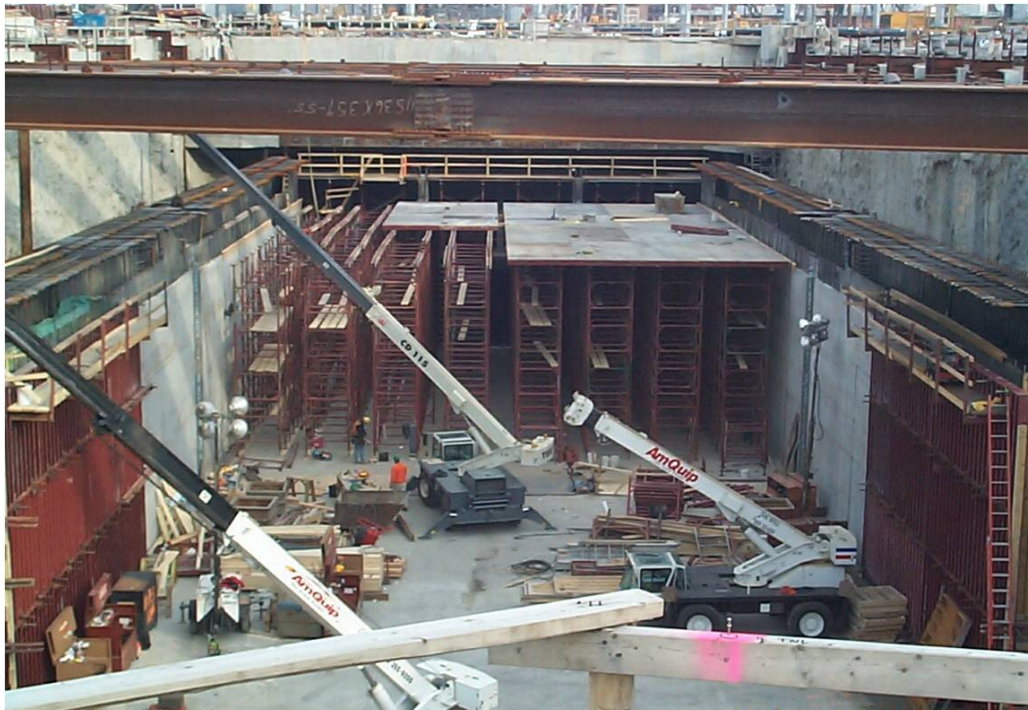
Figure 12-4 Tunnel Structure Construction Operation
