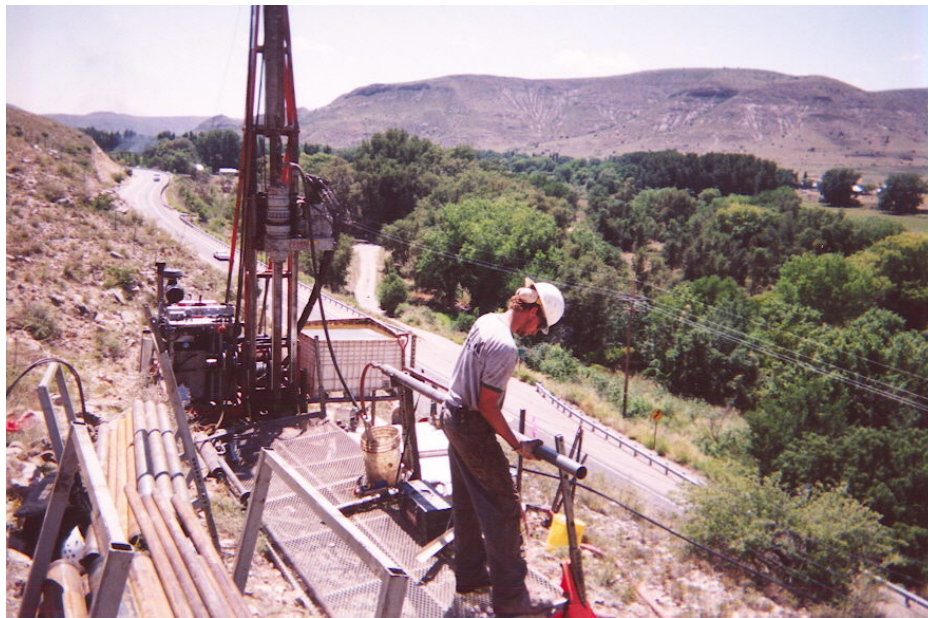
Figure 3-5 Vertical Test Boring/Rock Coring on a Steep Slope
