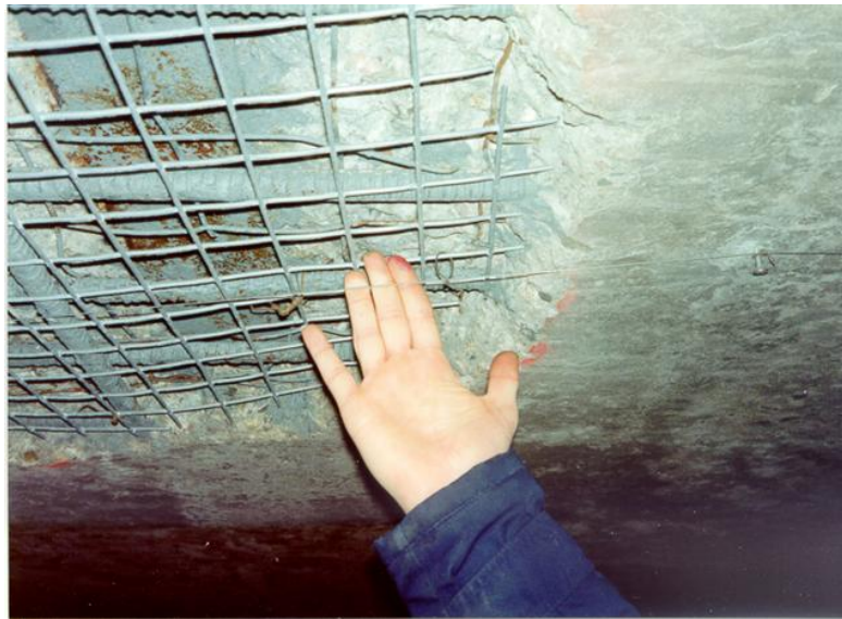
Figure 16-12 Reinforcing Steel for Repair, Sumner Tunnel Boston
