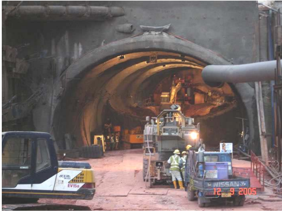
Figure 9-13 Soft Ground SEM Excavation Tunnel Using Backhoes (Fort Canning Tunnel, Singapore)
