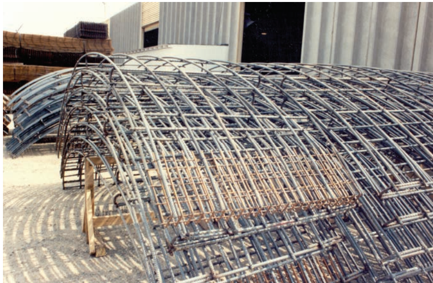
Figure 10-10 Steel Cage for Precast Segments for Two-Pass Lining
