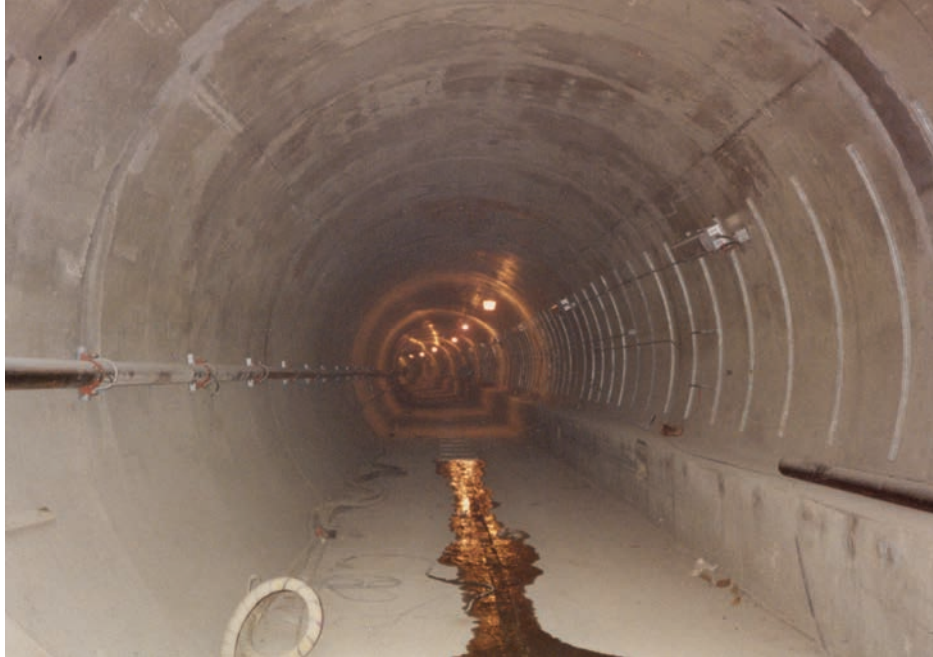
Figure 10-6 Cast-In-Place Concrete Lining, Washington DC
