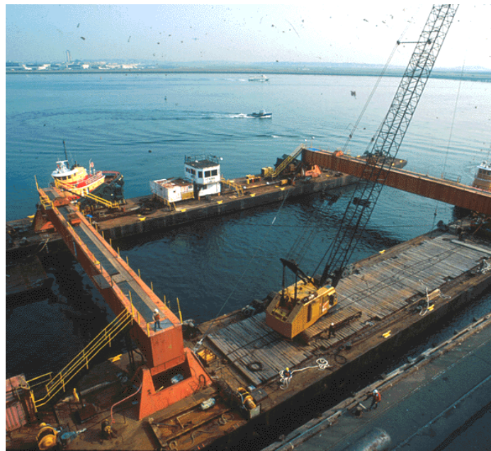
Figure 11-14 Catamaran Lay Barge
