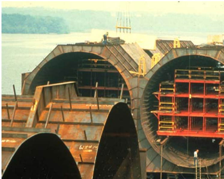
Figure 11-6 Fort McHenry Tunnel, Baltimore
