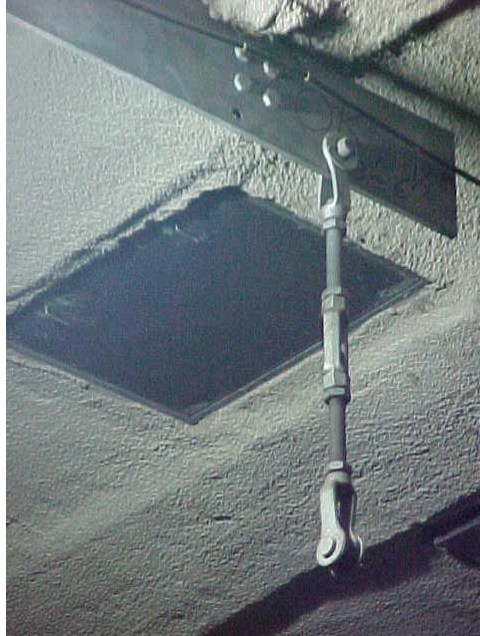
Figure 16-22 Typical Replacement Hanger Hardware
