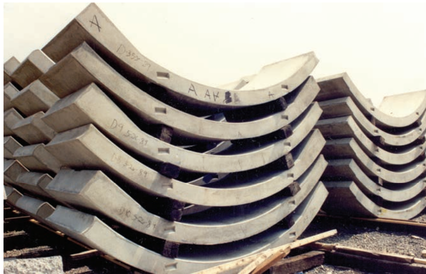
Figure 10-9 Stacked Precast Segments for Two-Pass Lining
