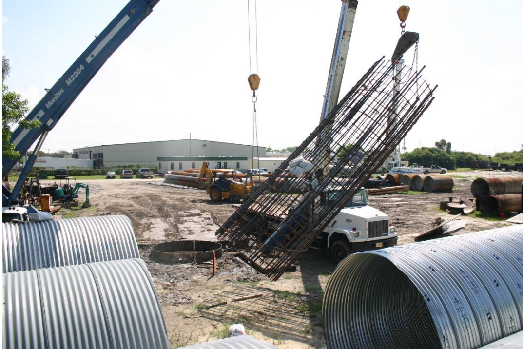
Figure 25. Photo. Picking of reinforcement cage for voided shaft.
