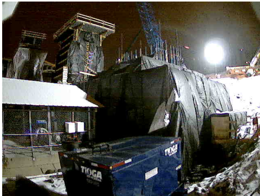
Figure 80. Photo. Interior column lift 2 formwork placement.
