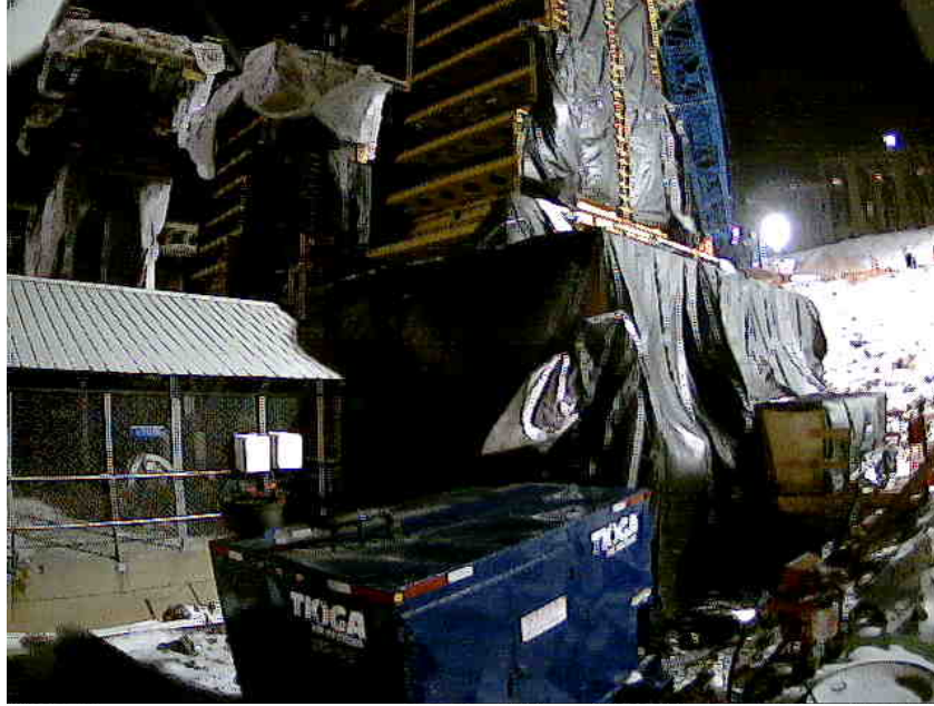
Figure 81. Photo. Exterior column lift 2 formwork placement.
