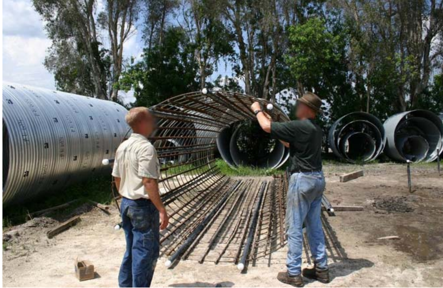
Figure 19. Photo. Voided shaft reinforcement cage instrumentation.
