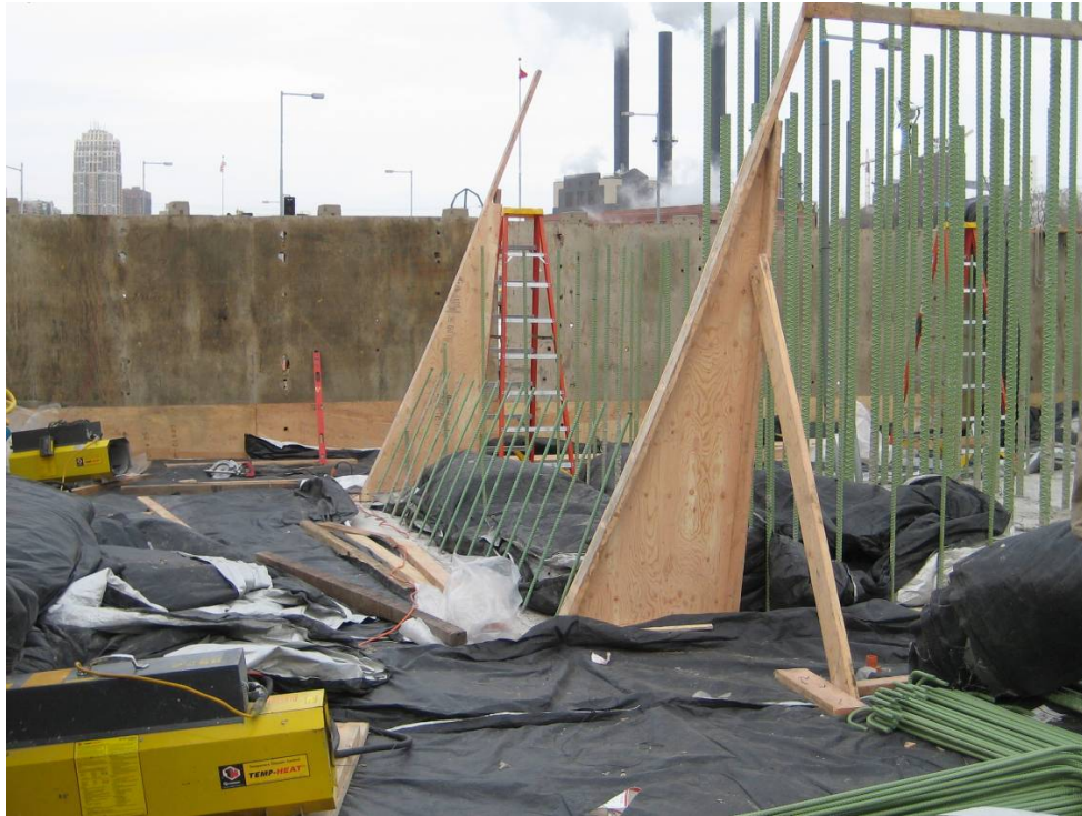
Figure 69. Photo. Reinforcement for first column pour for I-35W bridge columns.
