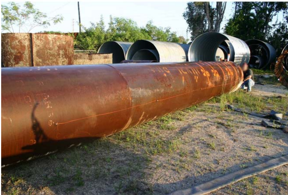
Figure 22. Photo. Voided shaft TCs on outside of center casing.
