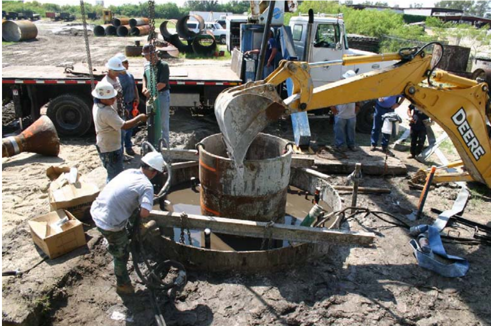
Figure 30. Photo. Holding of central casing steady for voided shaft.
