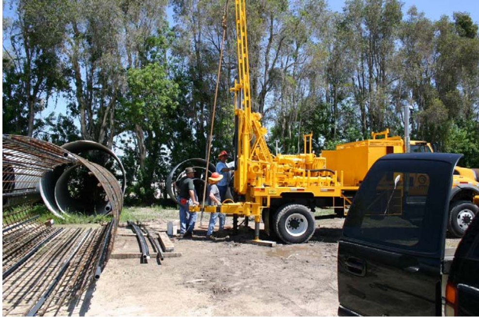
Figure 23. Photo. Voided shaft ground monitoring tube installation.
