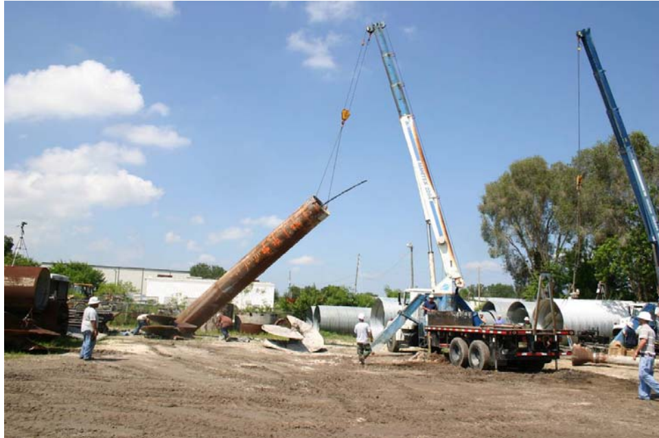
Figure 28. Photo. Picking of central casing for voided shaft.
