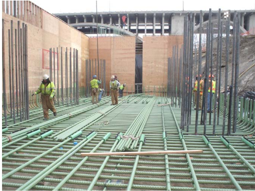
Figure 53. Photo. Lower layer of pier footing reinforcement for I-35W bridge.
