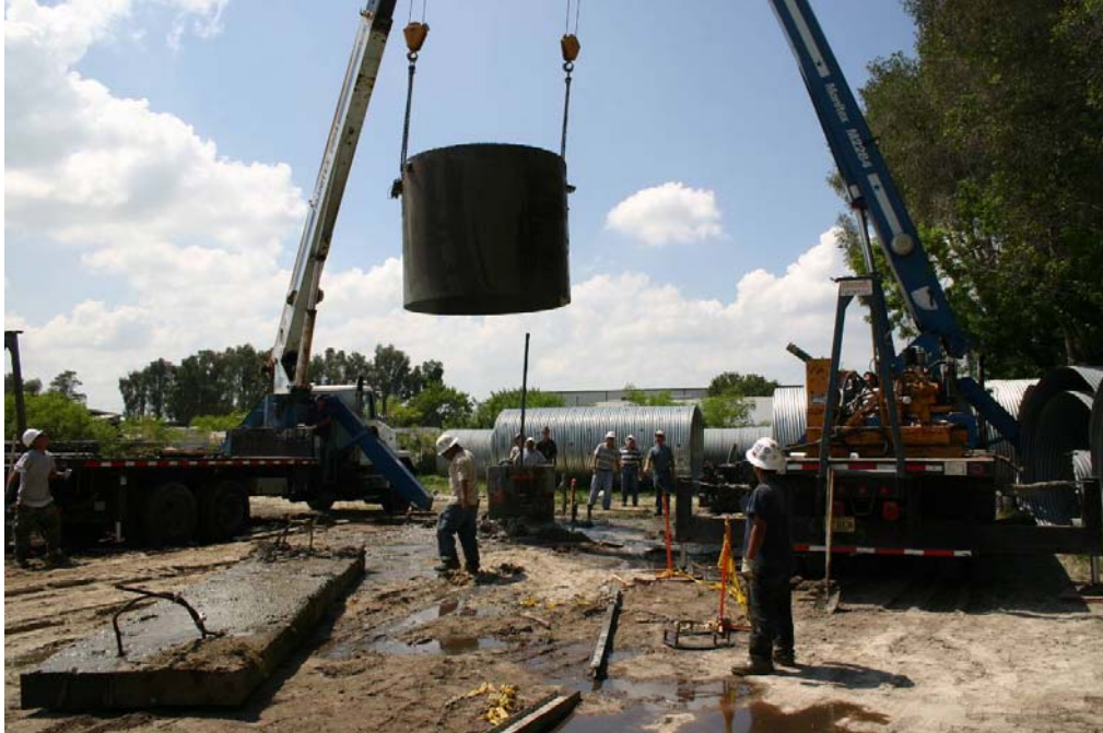
Figure 32. Photo. Voided shaft outer steel casing removal.
