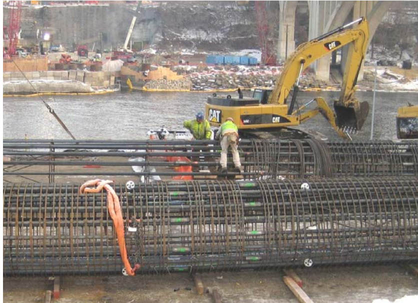
Figure 47. Photo. I-35W bridge shaft reinforcement cage construction.
