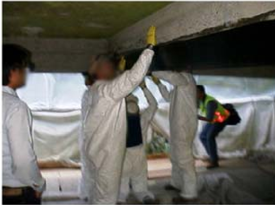
Figure 12. Photo. FRP wrap installation on bridge superstructure. (5)
