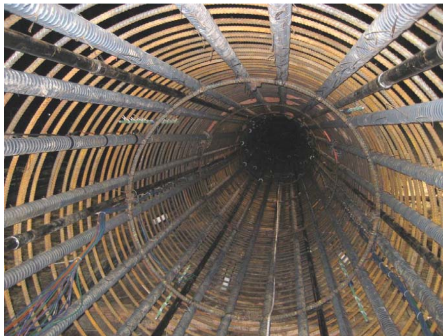
Figure 49. Photo. Cable bundles in reinforcement cage for I-35W bridge.
