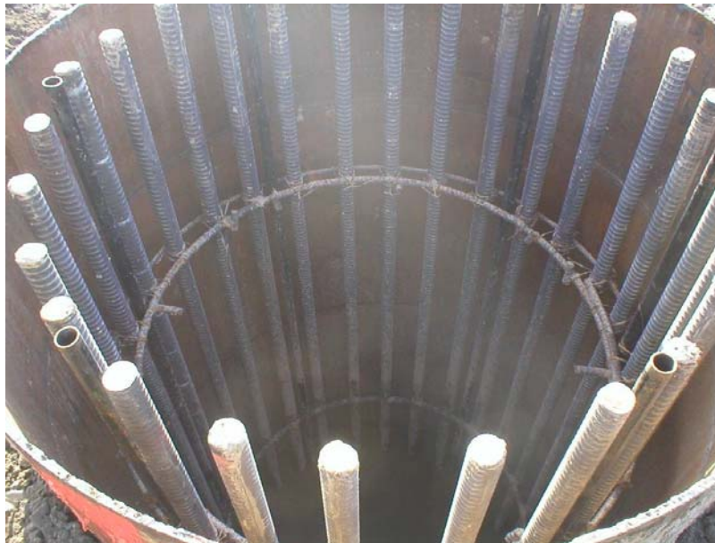
Figure 50. Photo. Top section of drilled shaft for I-35W bridge.
