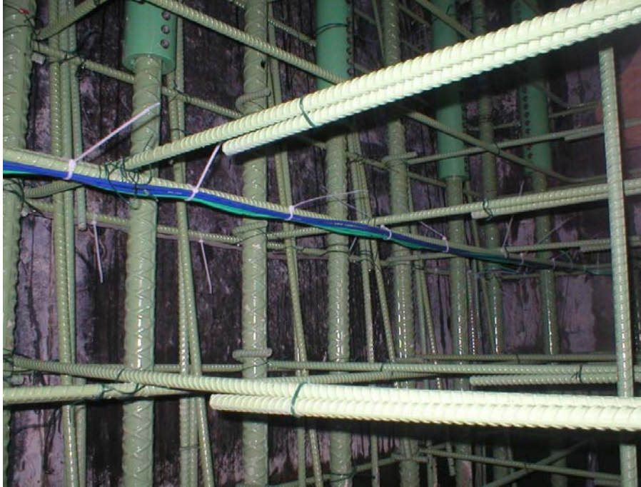
Figure 73. Photo. Gauge wires tied and secured in column of I-35W bridge.
