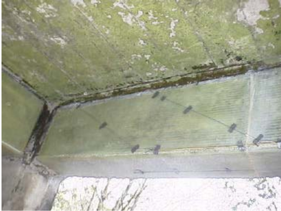
Figure 14. Photo. FOS installation over FRP wrap on bridge superstructure. (5)
