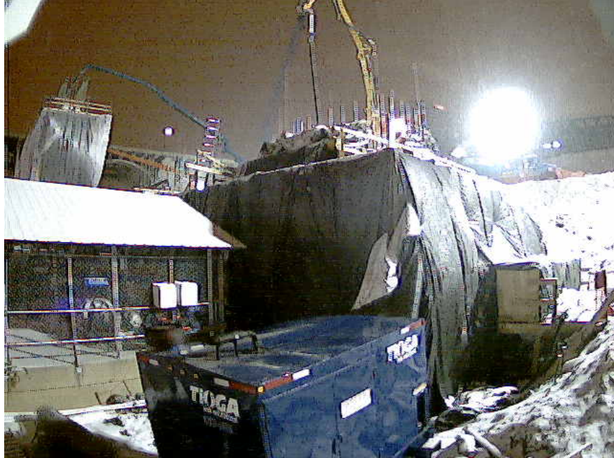
Figure 79. Photo. Lift 1 column concrete placement.
