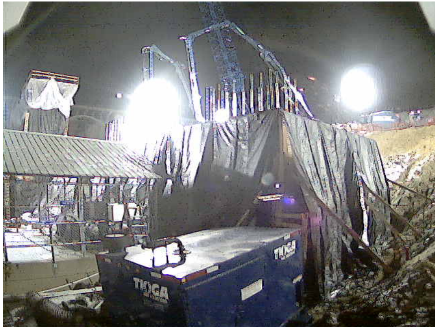
Figure 78. Photo. Pier footing concrete placement.
