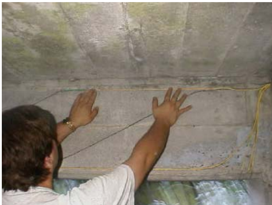
Figure 13. Photo. FOS installation on bridge superstructure. (5)
