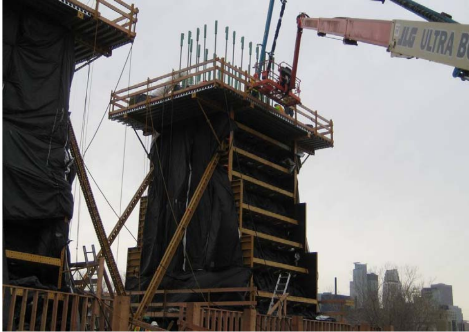
Figure 70. Photo. Reinforcement at midsection of columns for I-35W bridge.
