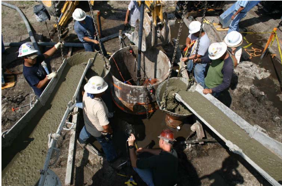
Figure 31. Photo. Double tremie concrete placement of voided shaft.
