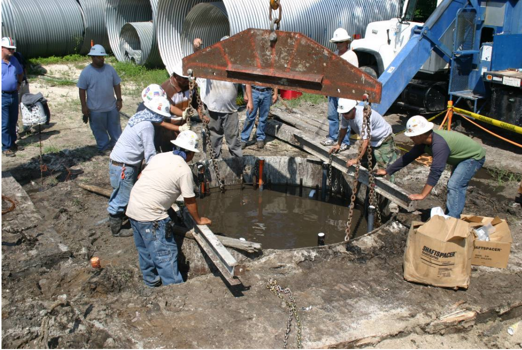
Figure 27. Photo. Hanging of reinforcement cage for voided shaft.
