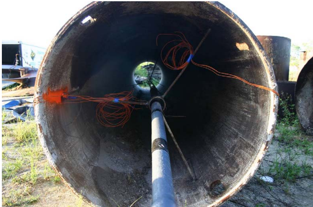
Figure 21. Photo. Voided shaft TCs installed in center casing.
