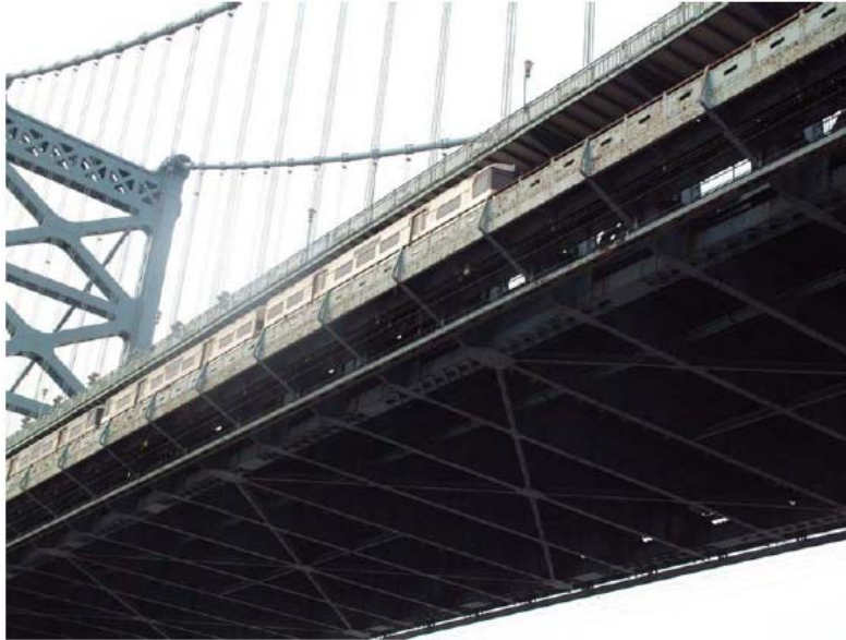
Figure 9. Photo. Train crossing bridge causing a strain event. (2)
