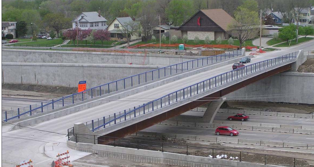
Figure 16. Photo. East 12th Street bridge in Des Moines, IA. (6)
