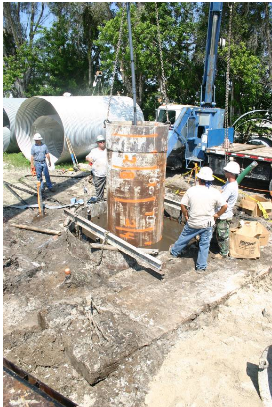
Figure 29. Photo. Placement of central casing for voided shaft.
