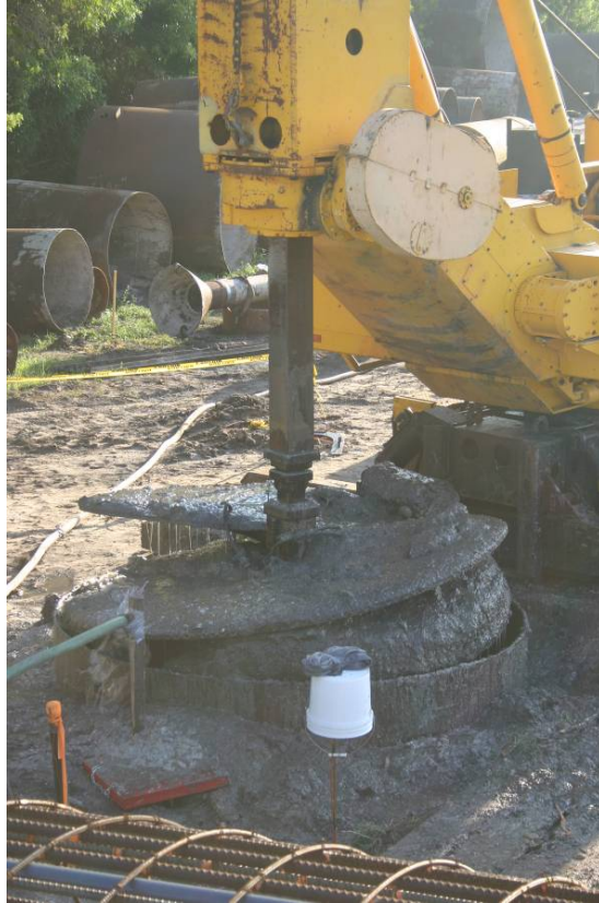
Figure 24. Photo. Excavation for voided shaft.
