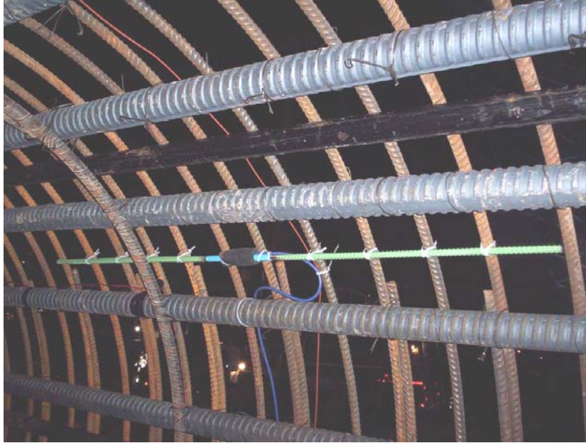
Figure 67. Photo. VW gauge installed in shaft reinforcement cage.
