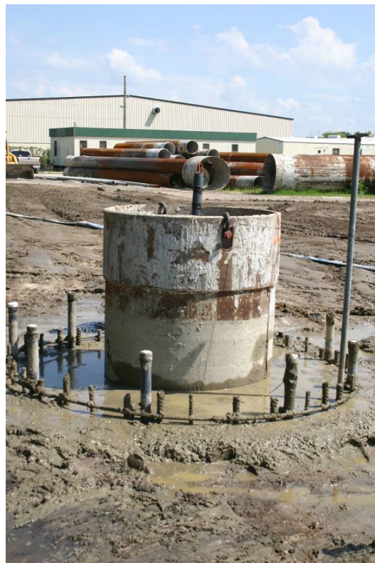
Figure 33. Photo. Final voided shaft at ground level.
