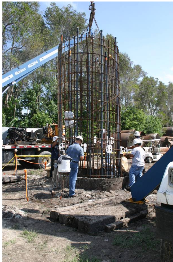
Figure 26. Photo. Placement of reinforcement cage for voided shaft.
