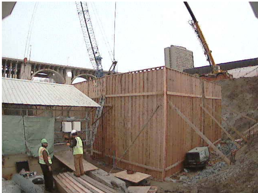
Figure 58. Photo. Sample camera shot from close-up camera on I-35W bridge.
