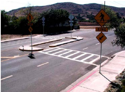
Figure A. Some crosswalks are angled to the right in the median. This is intended to facilitate a pedestrian's view of oncoming traffic before crossing the second half of the street.
