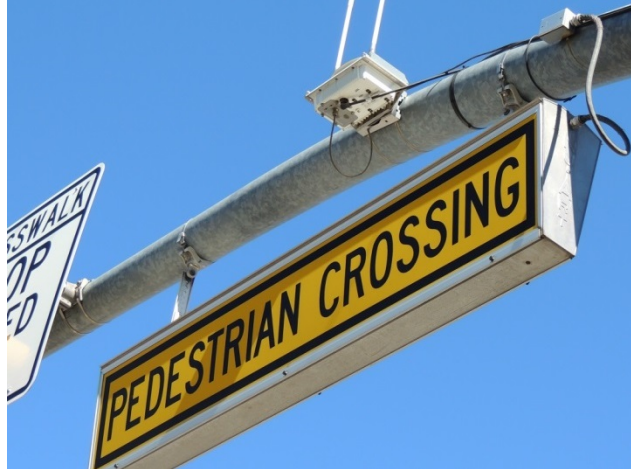
Figure 56. Photo. Example of internally illuminated sign used in Tucson, AZ.
