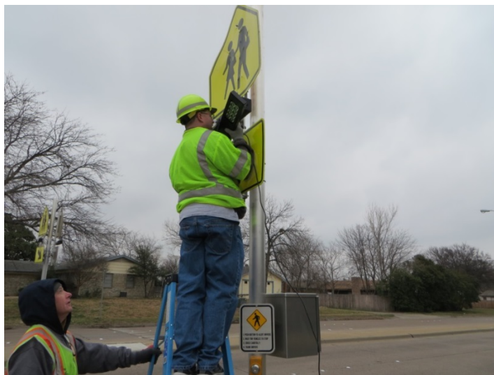
Figure 50. Photo. Installation of the light bar in field.
