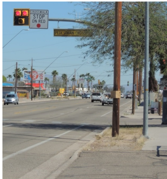
Figure 53. Photo. Example of PHB installation in Tucson, AZ.
