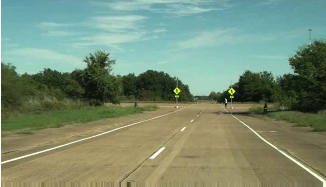
Figure 9. Photo. View at start of the driving video for the concluding survey for queries 1 and 2.
