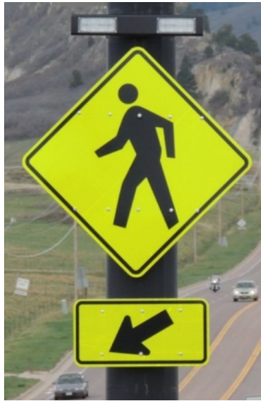
Figure 47. Photo. Example of RRFB placed above the sign.
