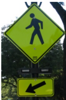
Figure 83. Photo. Rectangular beacons used at MK-07.
