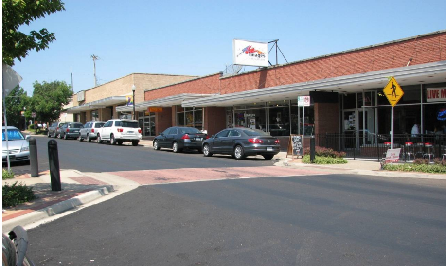
Figure 12. Photo. Unsignalized pedestrian crosswalk in Overland Park, KS.
