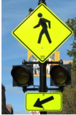
Figure 80. Photo. Circular beacons used at MK-04.
