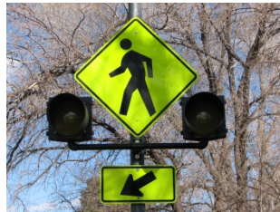
Figure 86. Photo. Circular beacons used at FG-02.
