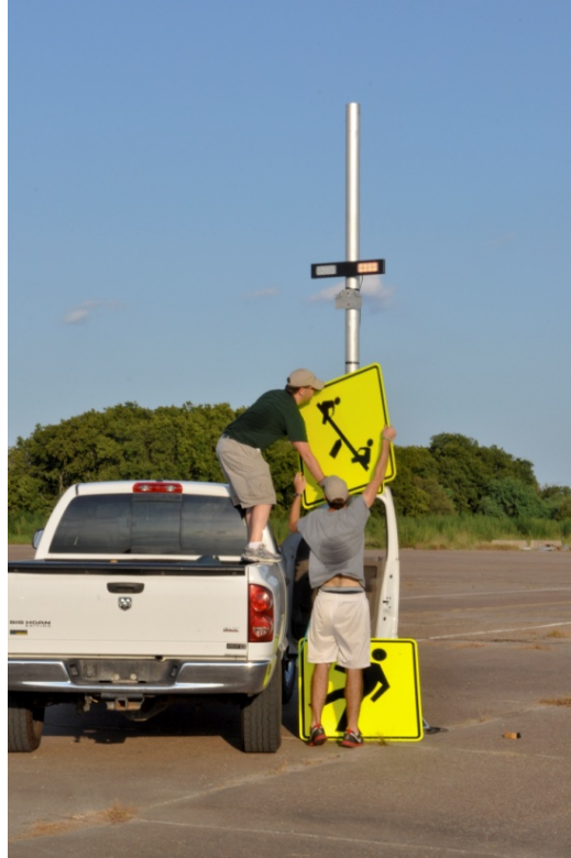
Figure 56. Photo. Another example of sign change.
