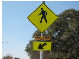
Figure 79. Photo. Rectangular beacons used at AU-02.
