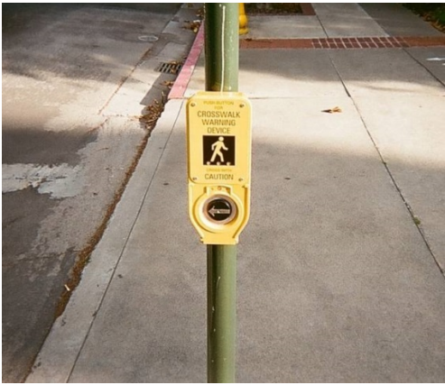
Figure 10. Photo. Unsignalized pedestrian crosswalk in Stockton, CA, pedestrian pushbutton.
