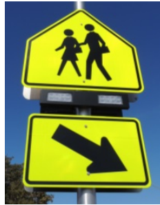
Figure 76. Photo. Rectangular beacons used at CS-01.
