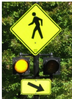
Figure 82. Photo. Circular beacons used at MK-06.
