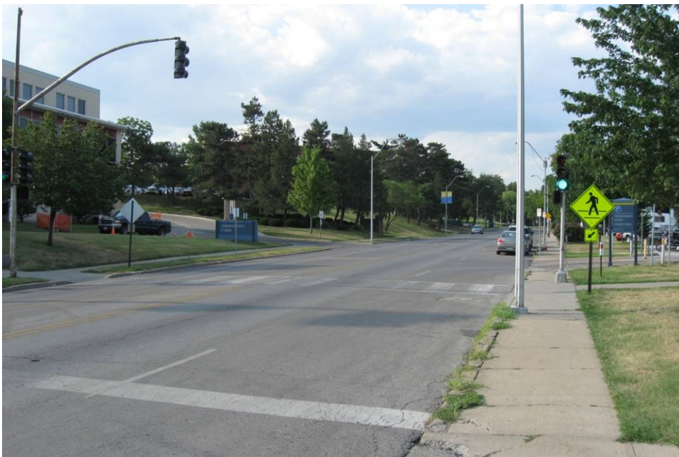
Figure 15. Photo. Another view of signalized pedestrian crosswalk in Kansas City, MO.
