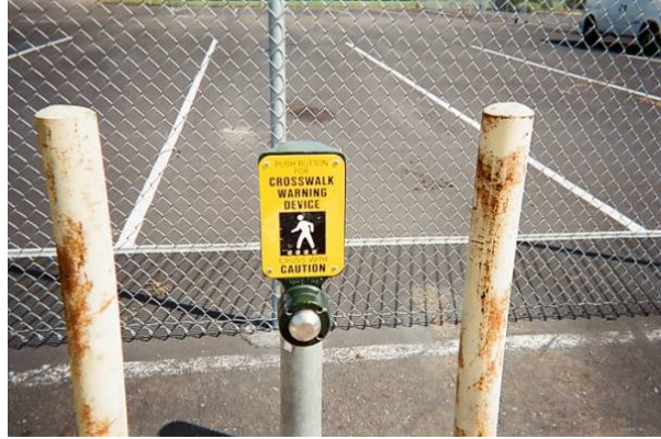
Figure 7. Photo. Unsignalized pedestrian crosswalk in Folsom, CA, pedestrian pushbutton.
