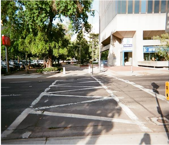
Figure 9. Photo. Unsignalized pedestrian crosswalk in Stockton, CA, pedestrian view.
