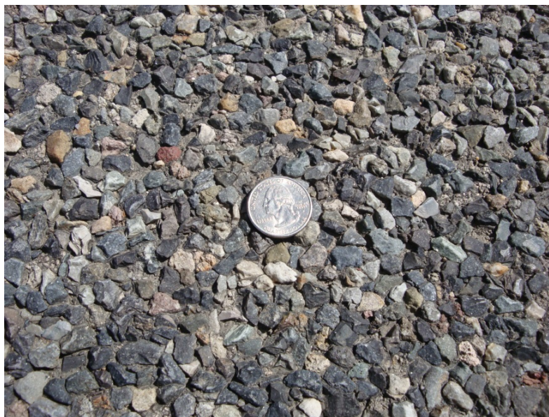
Figure 8. Photo. Placement of a chip seal (top) and surface texture of a single layer chip seal (bottom). (36)
