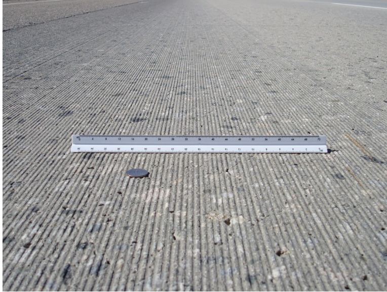
Figure 11. Photo. Diamond ground concrete pavement surface.
