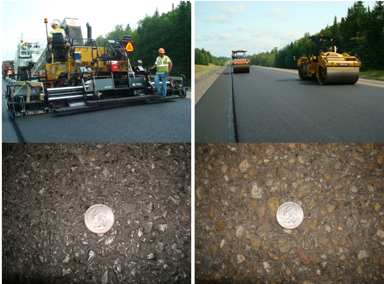
Figure 5. Photo. Placement of thin asphalt overlay (top) and surface texture of new (bottom left) and worn (bottom right) dense graded asphalt surfaces.
