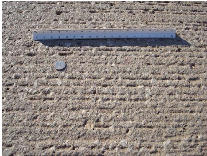
Figure 14. Photo. Shotblast asphalt pavement (top) and concrete pavement (bottom).
