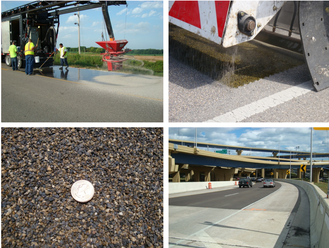
Figure 16. Photo. Installation of HFS (top) and finished surfaces (bottom).
