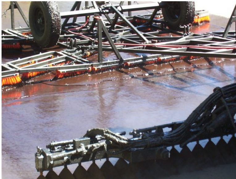
Figure 15. Photo. Emulsion material is scrubbed into the pavement surface for a scrub seal surface treatment. (41)
