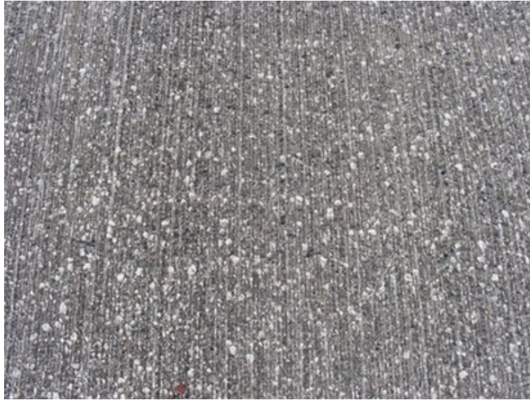
Figure 13. Photo. Micro-milled asphalt pavement surface. (40)
