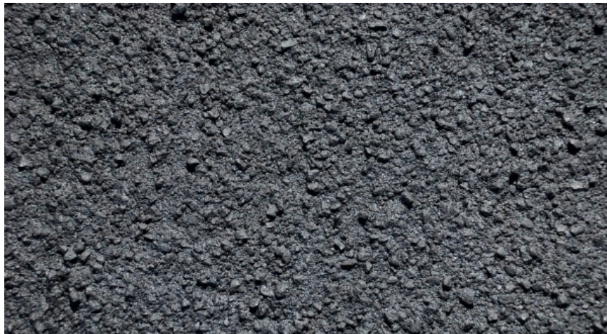
Figure 9. Photo. Placement of a slurry seal (top) and surface texture of a cured slurry seal (bottom). (37)
