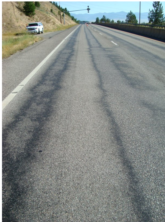
Figure 26. Photo. Example of wear in wheelpaths over time for chip seal treatments, reducing surface texture and friction.
