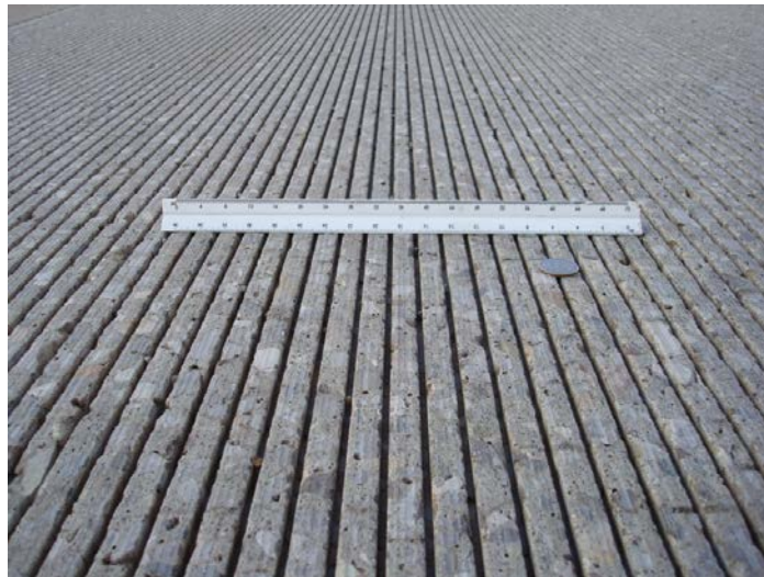
Figure 12. Photo. Grooved concrete pavement surface (top) and Next Generation Concrete Surface (bottom).
