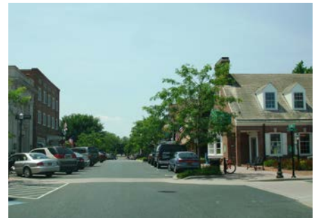
Small town Main Street districts can be revitalized with better sidewalks, curb extensions, crosswalks, parking, and landscaping (H.B. Rue).
