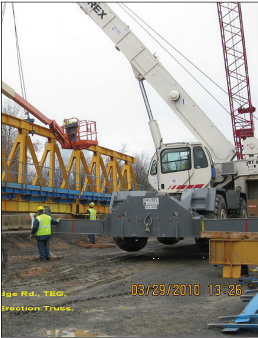
Dulles Corridor Metrorail Project construction, Northern Virginia
