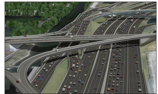
I-595 corridor roadway improvements.
