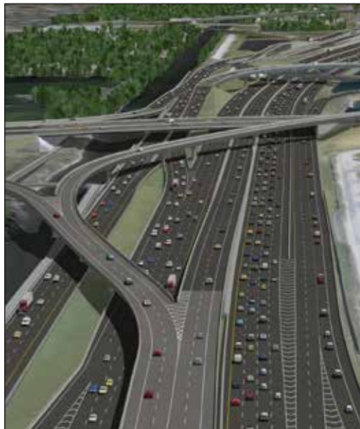
I-595 corridor roadway improvements
