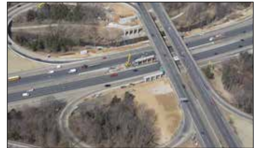
I-495 Capital Beltway high-occupancy toll lanes
