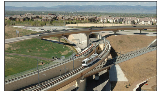
The T-Rex Project was delivered rapidly, thanks in part to early approval of funding.
