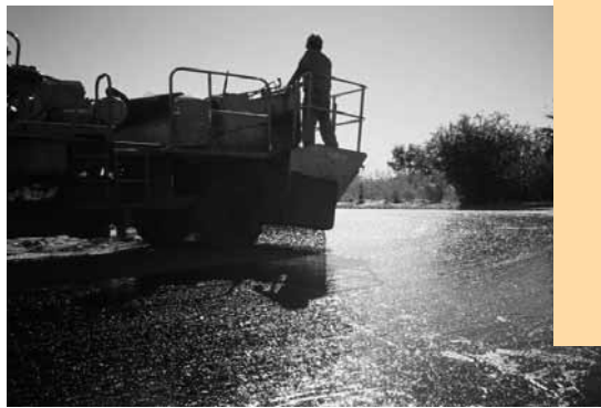
FHWA's new Transportation System Preservation Roadmap outlines and prioritizes pavement preservation and bridge preservation research needs. Preservation practices that can extend the service life of pavements and bridges, such as the chip seal for pavements shown here, are more important than ever as the Nation's infrastructure ages.
