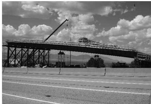
UDOT used SPMTs to remove the old 4500 South bridge (top). The superstructure of the new bridge was constructed offsite over a period of 4 months (bottom left). Following installation of the new bridge, I-215 reopened to traffic after a single weekend of work (bottom right).
