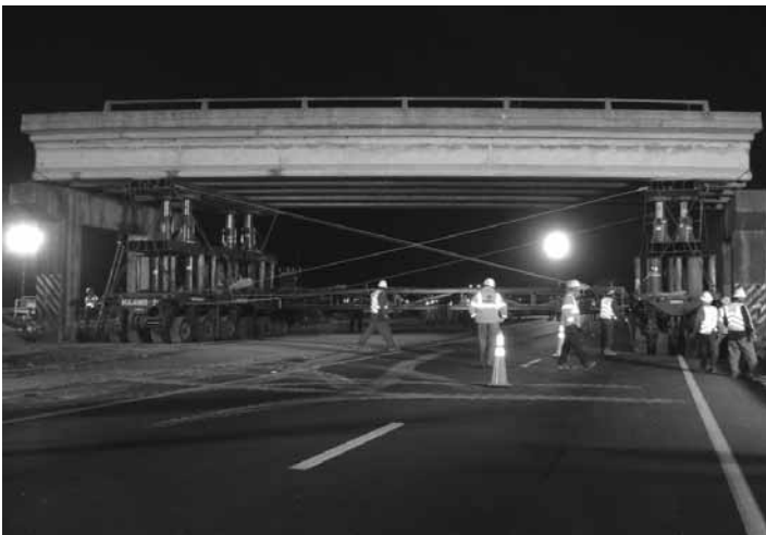
By using prefabricated bridge elements and SPMTs, the Florida Department of Transportation cut months off the project schedule for constructing the new Graves Avenue bridge in Volusia County in 2006.
