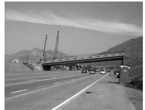
UDOT used SPMTs to remove the old 4500 South bridge (top). The superstructure of the new bridge was constructed offsite over a period of 4 months (bottom left). Following installation of the new bridge, I-215 reopened to traffic after a single weekend of work (bottom right).
