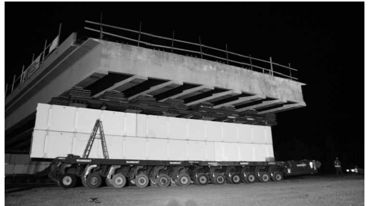
By using prefabricated bridge elements and SPMTs, the Florida Department of Transportation cut months off the project schedule for constructing the new Graves Avenue bridge in Volusia County in 2006.
