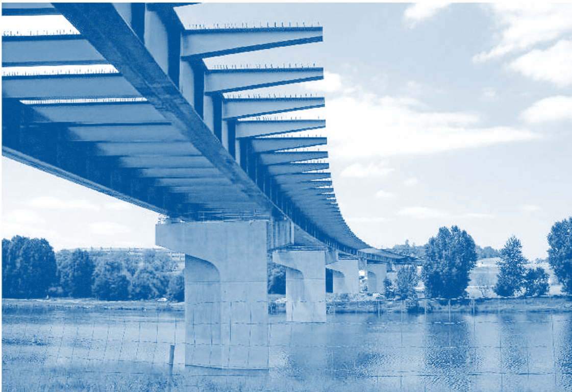
Figure 13. Typical two-girder system in Europe.
