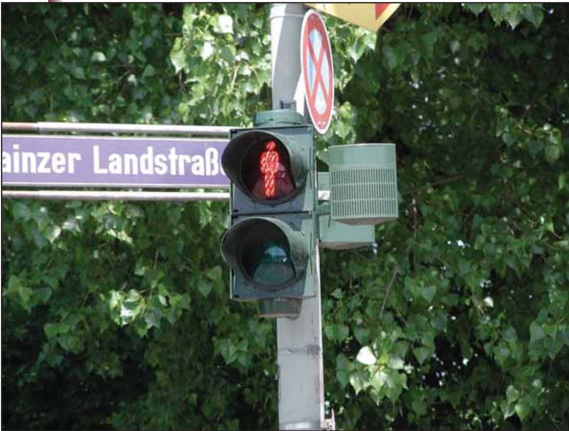
Figure 3-3. Audible pedestrian signal head in Germany.
