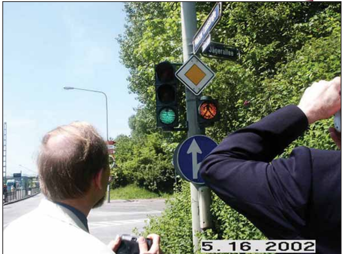
Figure 4-7. Supplemental signal warning right-turning motorists about pedestrians.
