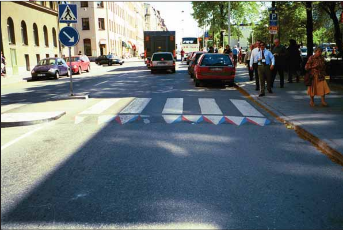
Figure 4-5. Virtually raised crosswalks in Sweden.
