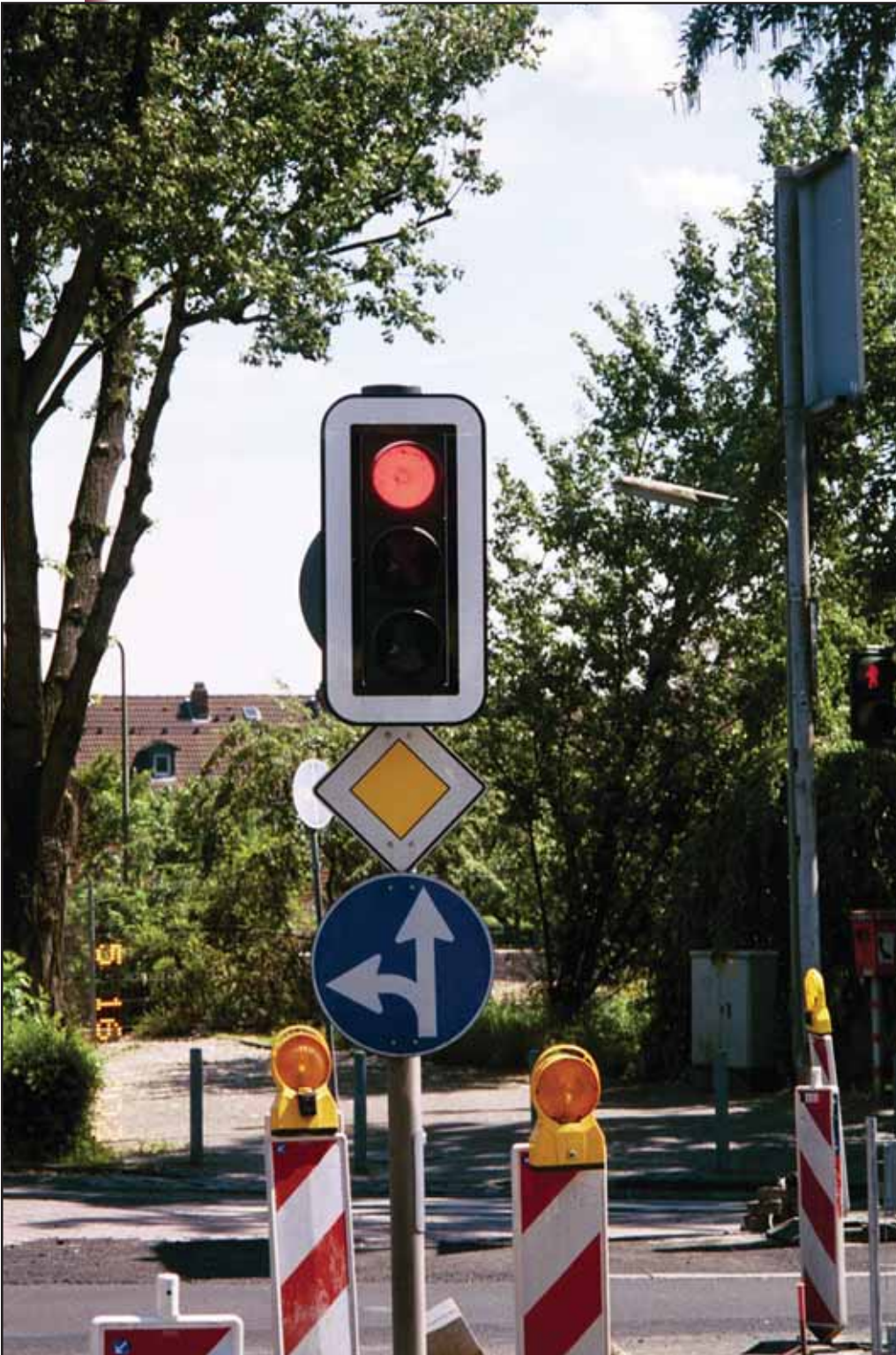
Figure 4-6. Traffic signal with back plate in Germany.
