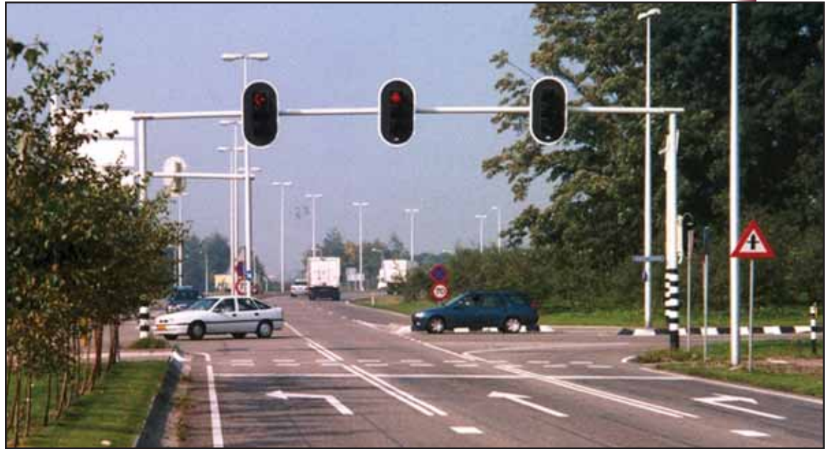
Figure 4-11. Large back-plate bordered by white stripe.
