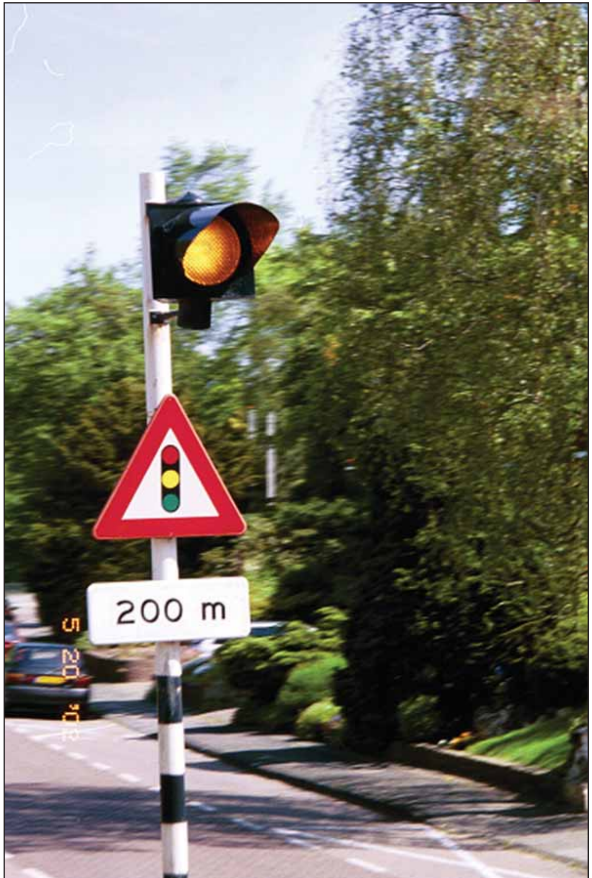
Figure 4-9. "Signal ahead" warning sign in the Netherlands.
