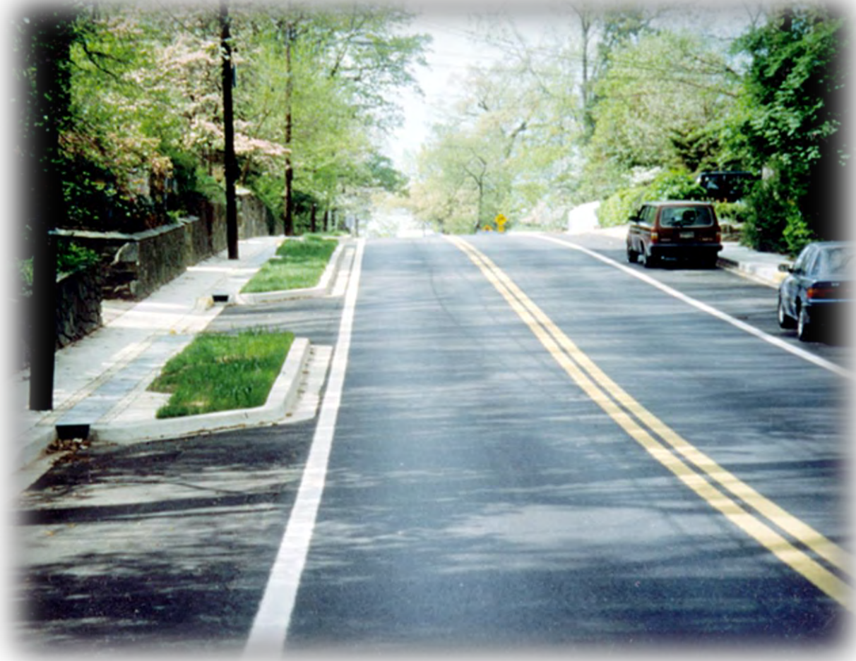
Photo: Typical example of a two lane transportation project with sidewalks, curb landscaping, and street parking.
