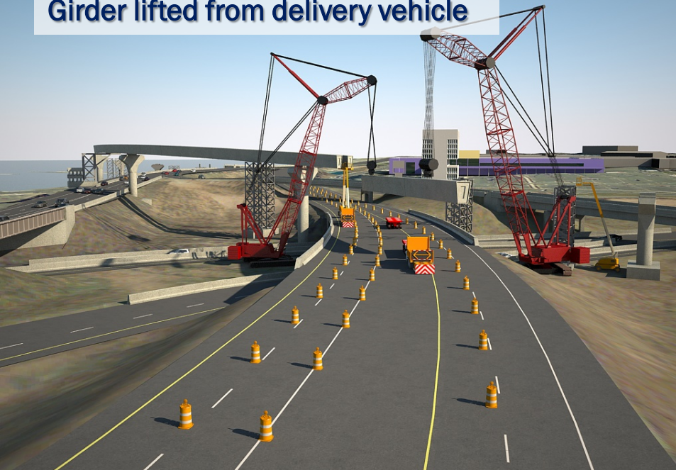
Crane rigging detached Right lanes opened to traffic
