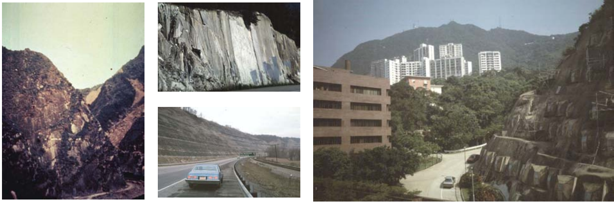
Figure 3-23. Rock Formations Showing Joints, Cut Slopes, Planes, and Stabilization Measures.
