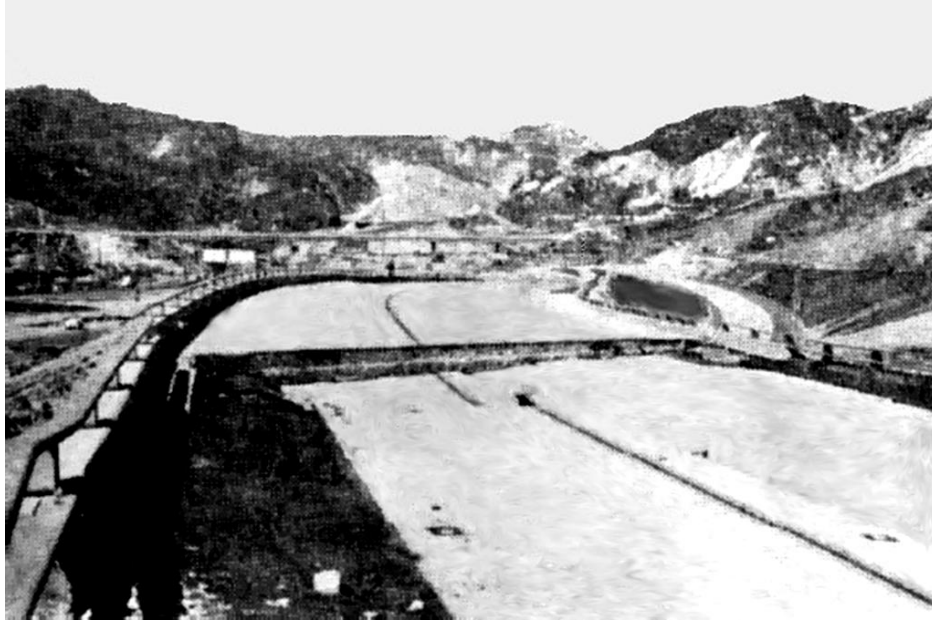
Figure 1-9 Settlement of Abutment Embankment Fill in the 1971 San Fernando Earthquake (FHWA, 2004)
