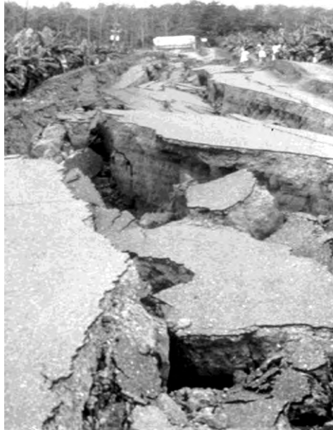
Figure 7-10 Disrupted Fill and Pavement due to Liquefaction at the Approach to the Highway 36 bridge Over Rio Estrella, Costa Rica, during 1991 Earthquake.
