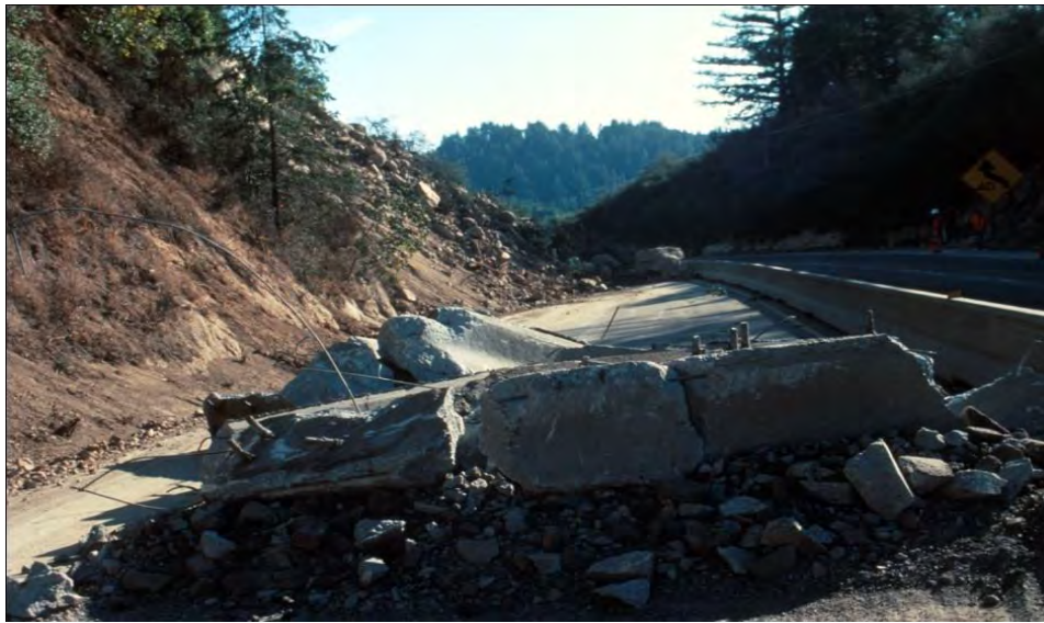
Figure 1-12 Landsliding Along SR-17 in the 1989 Loma Prieta Earthquake (USGS)
