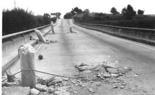
Figure 10-3 Piles Punched-Through the Deck Slab in the Collapsed Struve Slough Bridge (EERI, 1990)
