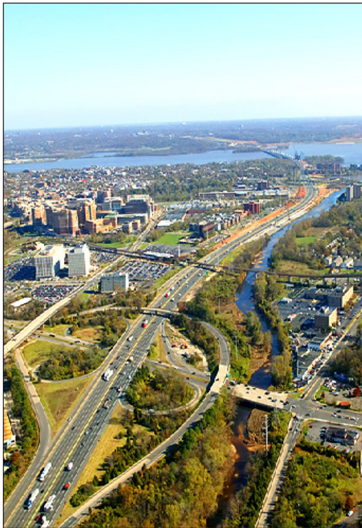
Capital Beltway high-occupancy toll lanes was the first project to utilize PABs.
