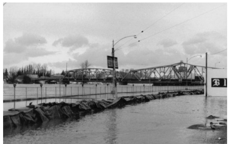
Sandbag Revetment during the 1980 flood event
