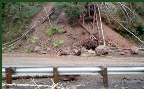
Debris from a landslide covered Oregon Highway 6 in March 2014. Photo credit: Oregon Department of Transportation
