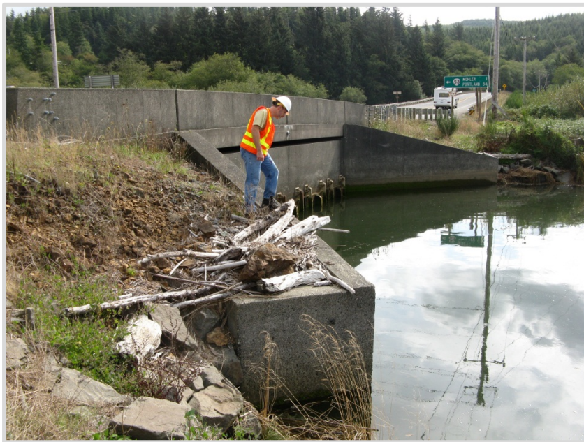
Inspecting the bridge wing wall at Gallagher Slough.
