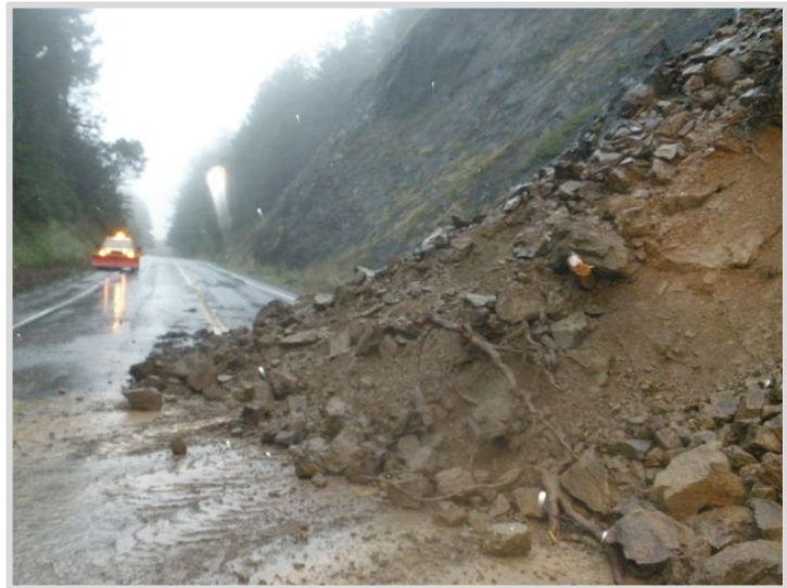
More than 400 yards of rocks and mud slid onto U.S. 101 south of Port Orford in March 2012.
