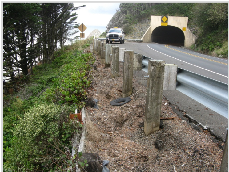
Northbound U.S. 101 at Arch Cape tunnel.
