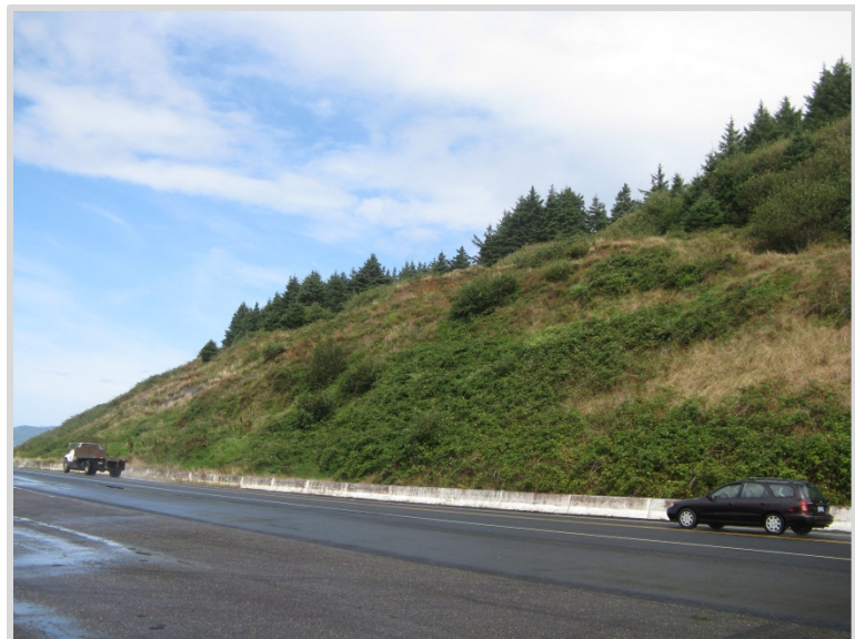
The Silverpoint landslide as seen from U.S. 101 south of Cannon Beach.
