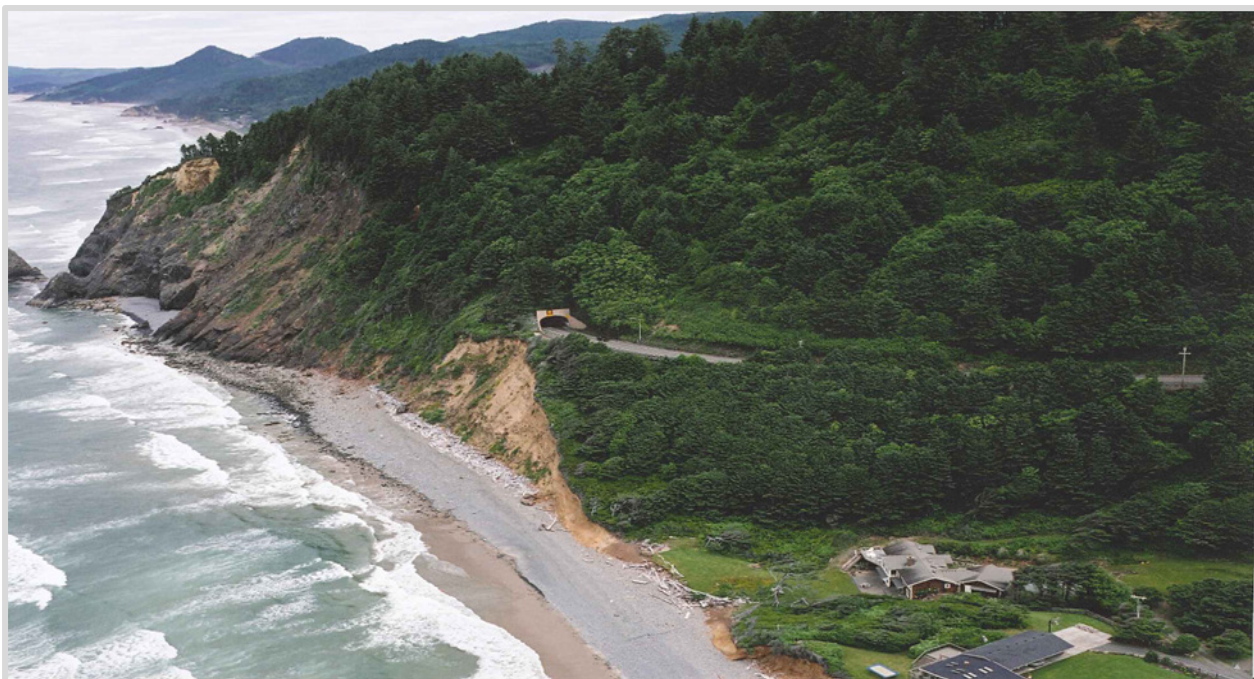
The view north to Arch Cape tunnel and coastal bluff.
