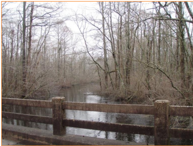
Figure 5-49. Structure 31 Facing Downstream Photo Source: (Maryland Environmental Services 2006)
