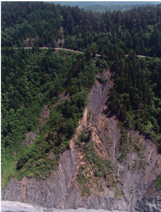
Figure 8: Gully Erosion at Last Chance Grade, Del Norte County
