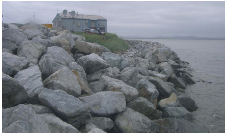
Figure 12: Kivalina's Rock Revetment 50
