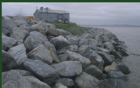
A rock revetment in Kivalina, Alaska. Photo credit: USACE
