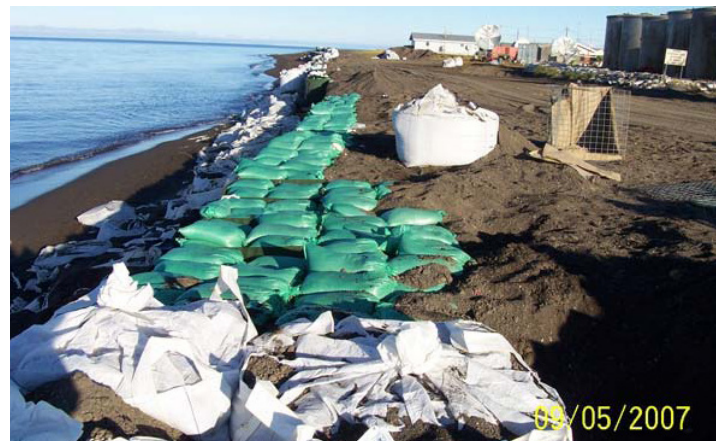
Figure 1: Kivalina's 2007 Revetment. Source: USACE
