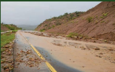
August 2014 flooding that closed part of Interstate 17. Photo credit: ADOT
