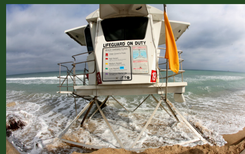
A flooded and damaged beach patrol tower. Photo credit: Art Seitz.
