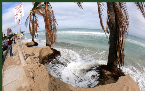
A severely eroded beach in South Florida. Photo credit: Art Seitz.
