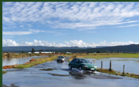
Flooding impacts to road. Photo credit: Aldaron Laird.
