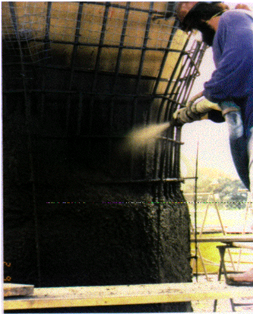
Nozzleman Applying Shotcrete
