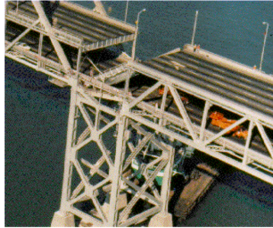
San Francisco-Oakland Bay Bridge
