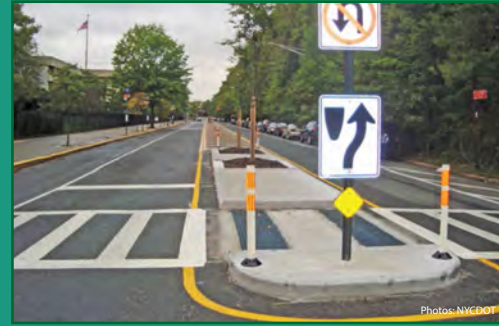
A pedestrian refuge island improves safety for pedestrians near Tottenville High School.
