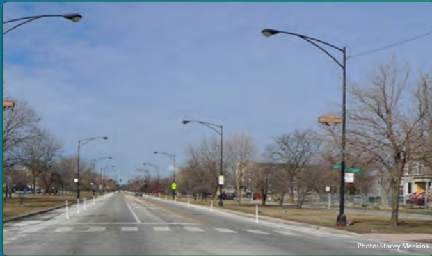
3-lane cross-section with bollard-separated bicycle lanes
