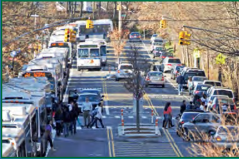
A Road Diet was installed along Luten Avenue to enhance safety for all road users.
