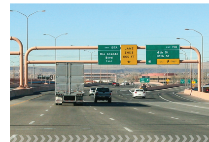
Assessing driver behavior near closely spaced interchange ramps. | Photo courtesy University of Utah
