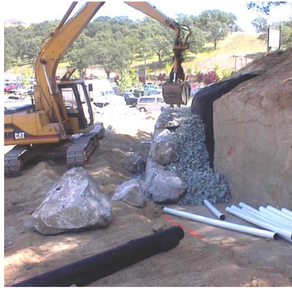
Figure 62. Photograph. Hydraulic excavator with a clamshell constructing a rockery.
