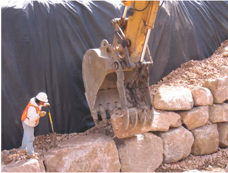
Figure 63. Photograph. Placement of facing rocks using an excavator with a “thumb.”
