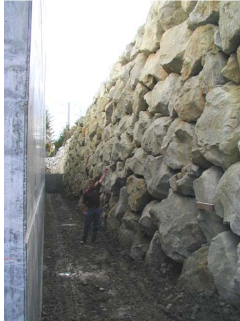
Figure 15. Photograph. Single-tier, 7.6-m (25-ft) rockery in Tacoma, Washington (Site 5).
