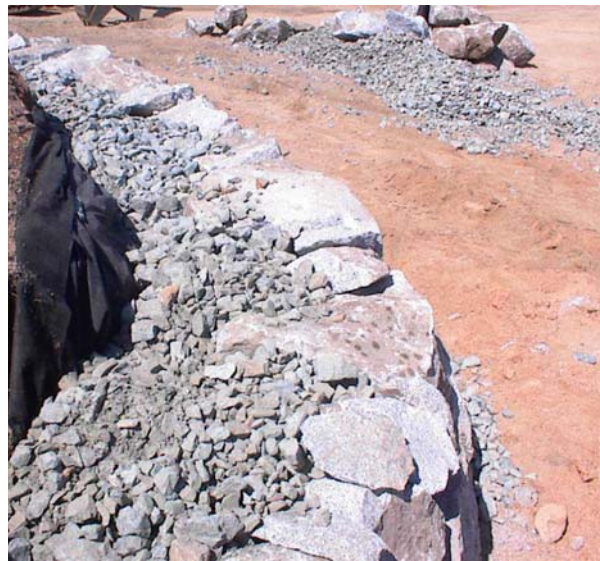
Figure 71. Photograph. Example of crushed rock placed behind rockery.
