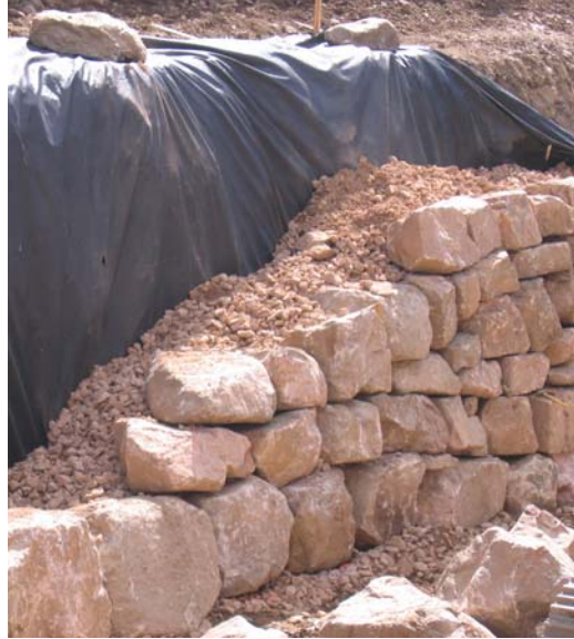
Figure 72. Photograph. Placement of drain blanket and non-woven geotextile behind rockery.
