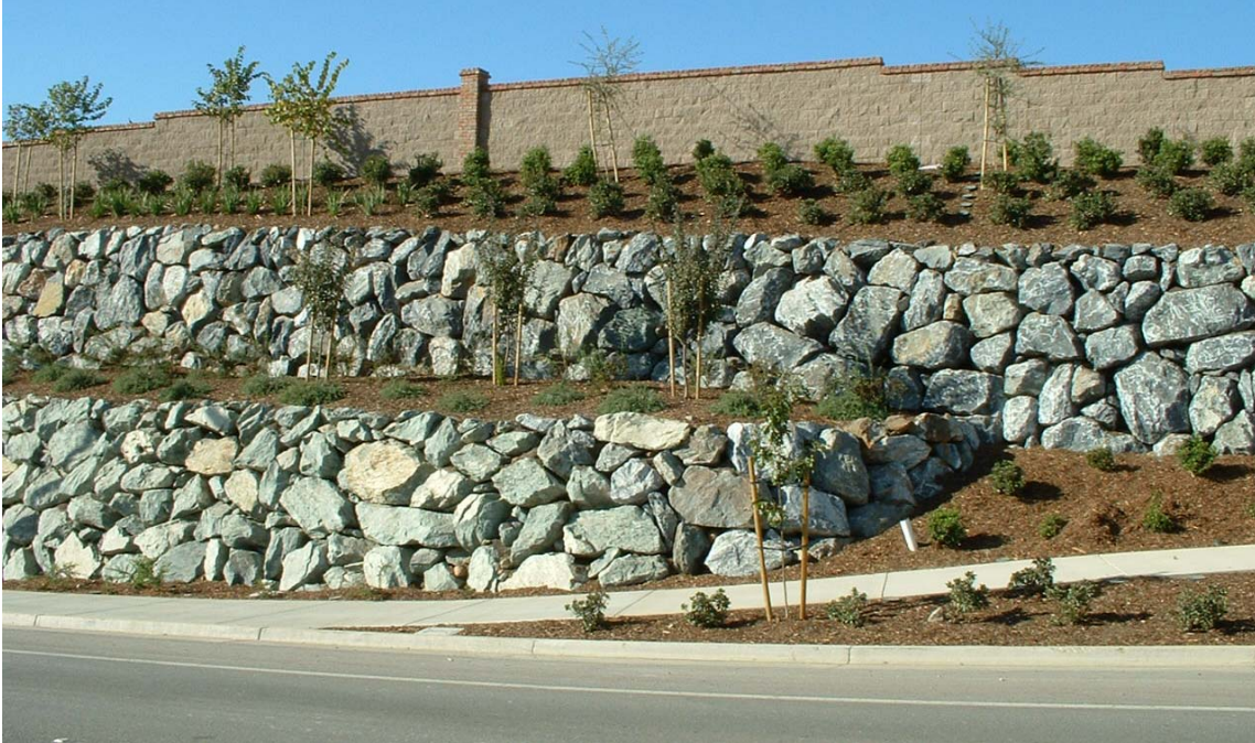
Figure 74. Photograph. Example of proper layout, interlock, and chinking of variable shape and size rocks.
